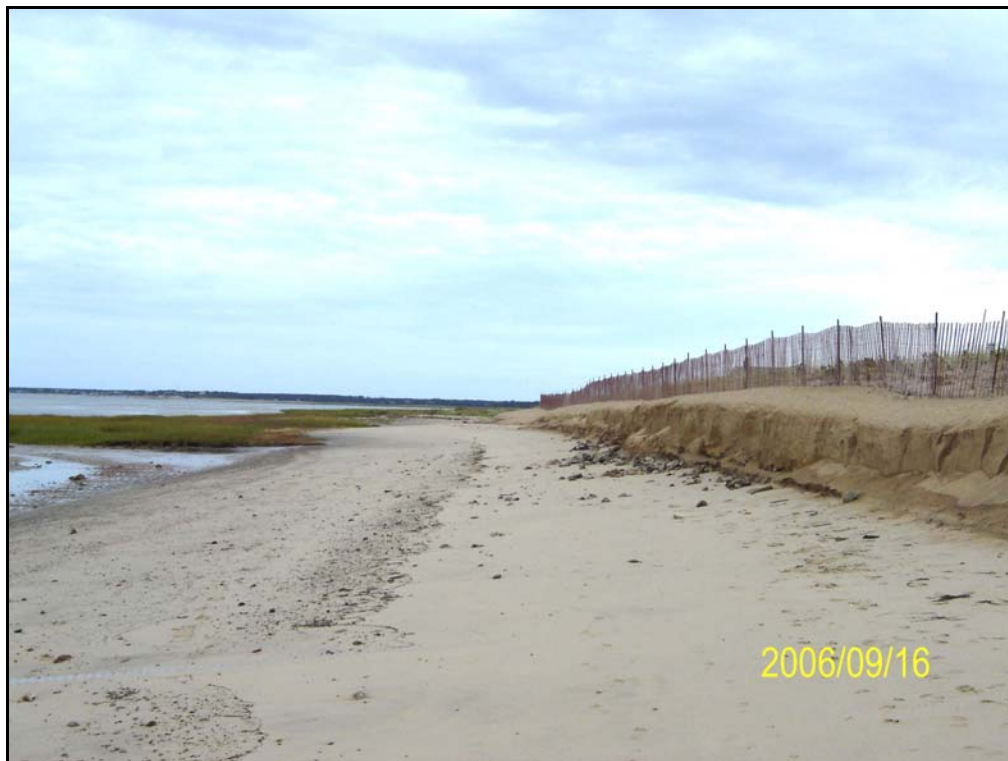
Figure 7. Coastal erosion causing the burial of a salt marsh at a dune restoration site. NAMSKAKET, ORLEANS
