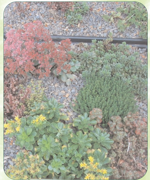
Close up of plantings on Boston's City Hall roof-top terrace. These mini gardens help hold and treat stormwater runoff.
