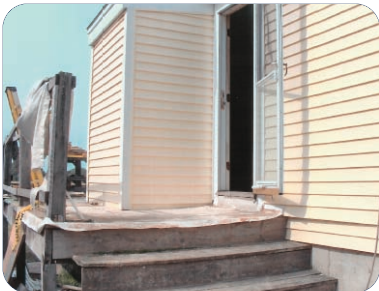
This small addition, built with FEMA assistance, holds a Quincy home's utilities and appliances above projected floodwaters. Thanks to innovative braces, the addition doesn't increase the building's footprint.
