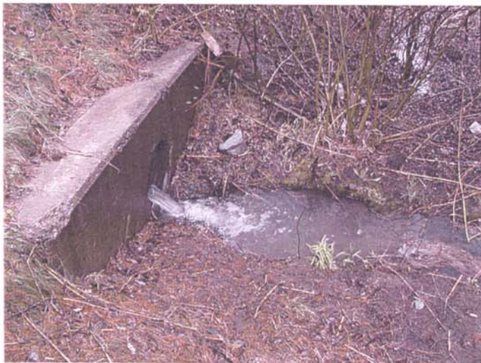
Figure 2-11: Discharge from catchbasin into the wetland at Cherry Hill site.
