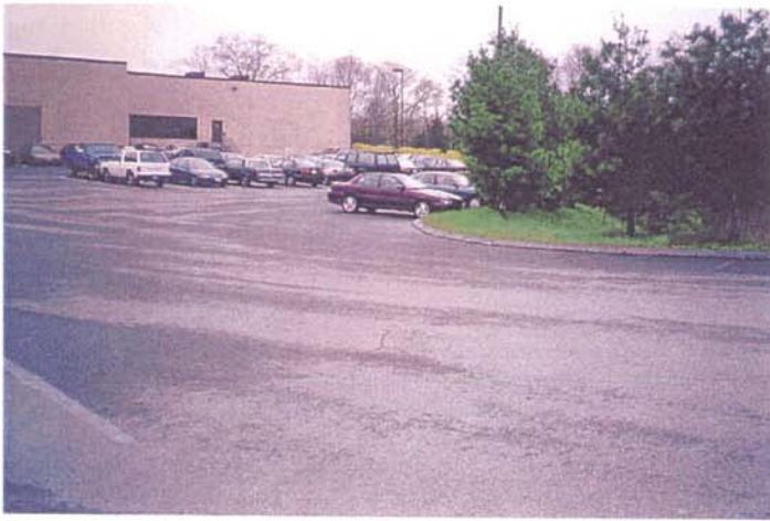
Figure 2-9: Part of the parking lot draining into the wetland.
