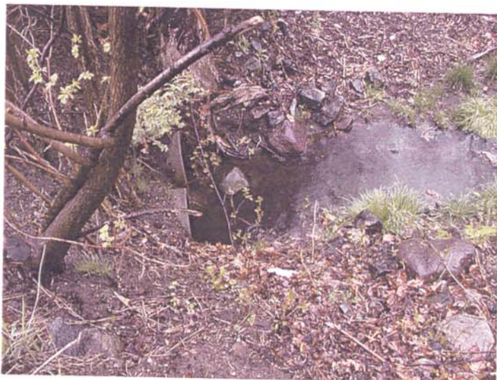
Figure 2-4: Sampling location at the Pinefield site. The location consists of two parallel, partially submerged 12" diameter drainage pipes.
