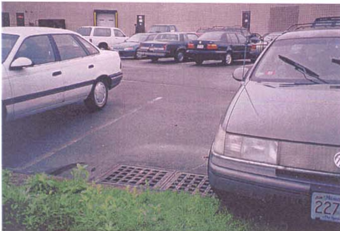
Figure 2-10: Manhole cover for catchbasin at parking lot at Cherry Hill site. The catchbasin overflows into the wetland.
