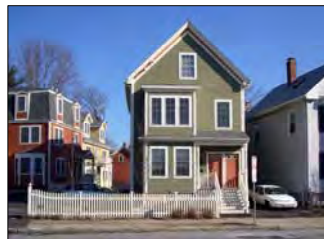
Two-family units should include raised ground floors, steep pitched roofs, and articulated facades or bay windows.
