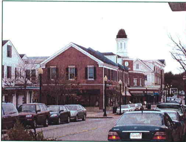
The series of buildings on the blocks above include a variety of roof lines, building materials and façade elements, but exhibit general consistency of fenestration patterns and proportions.
