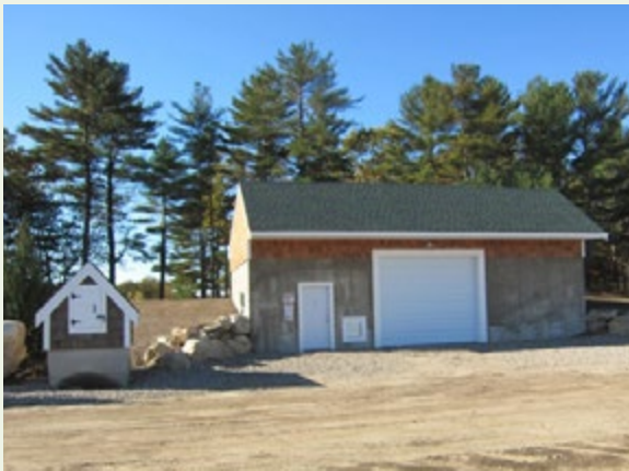
Pesticide Storage and Mixing Facility, Edgewood Bogs, Carver, MA
