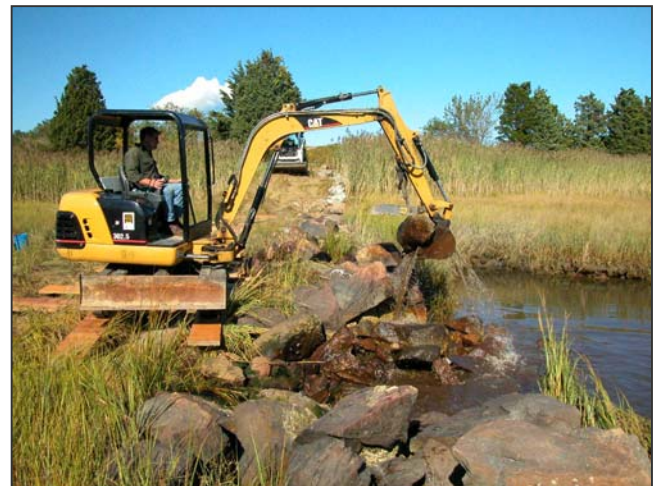
Figure 4. EMC sites before and during dike work to remove sections in channel.
