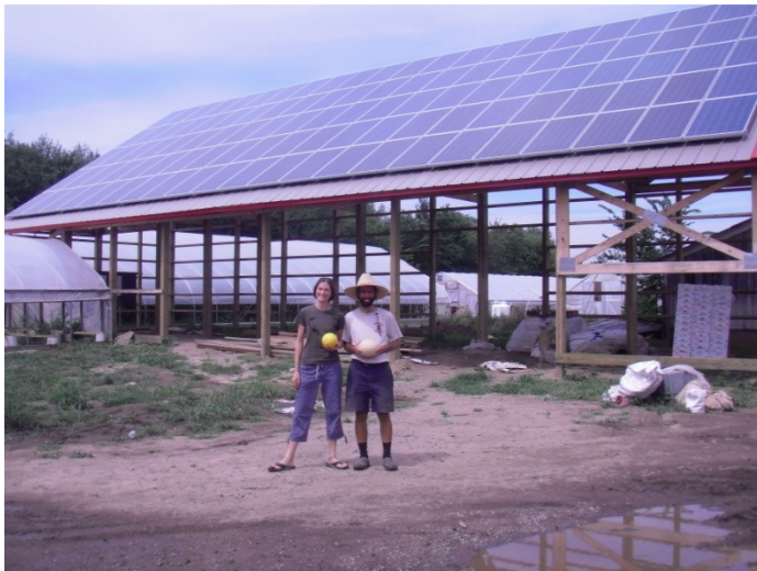
Figure Seven: 10KW PV System Red Fire Farm Granby
