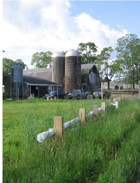
Figure One: Wastewater Treatment Strip
