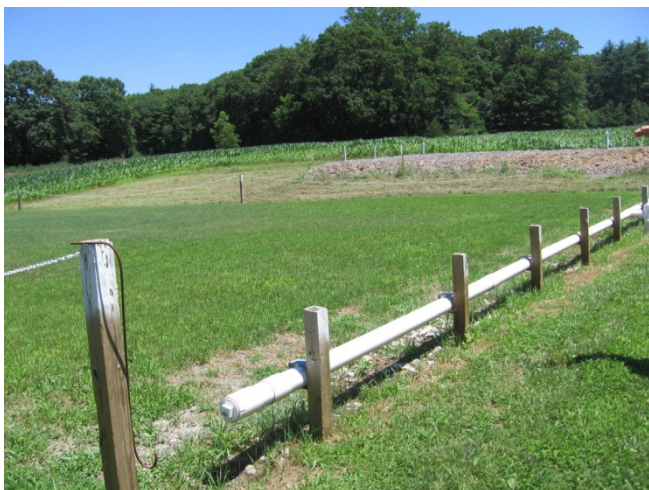
Figure Six: Vegetated Treatment Area and Bark Bed System, Great Brook Farm
