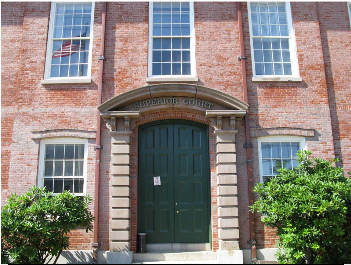
Newburyport Superior Courthouse Entrance
