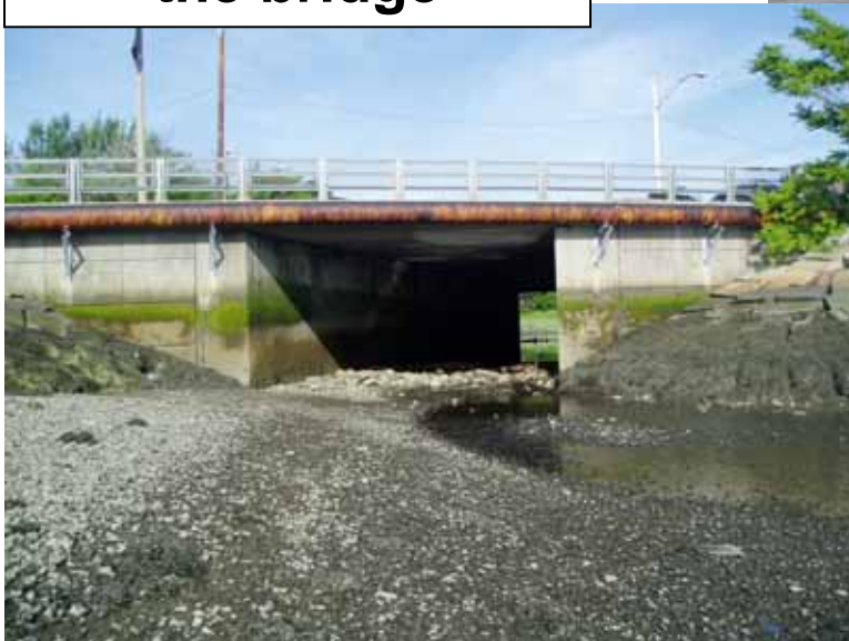
Looking west at the bridge
