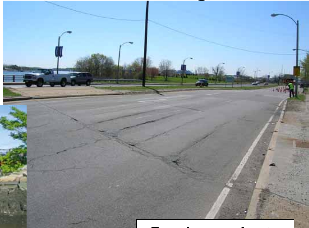
Roadway prior to recent overlay
