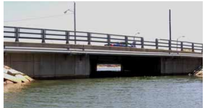
Morrissey Blvd. over Patten's Cove (Bonetti Memorial Bridge)
