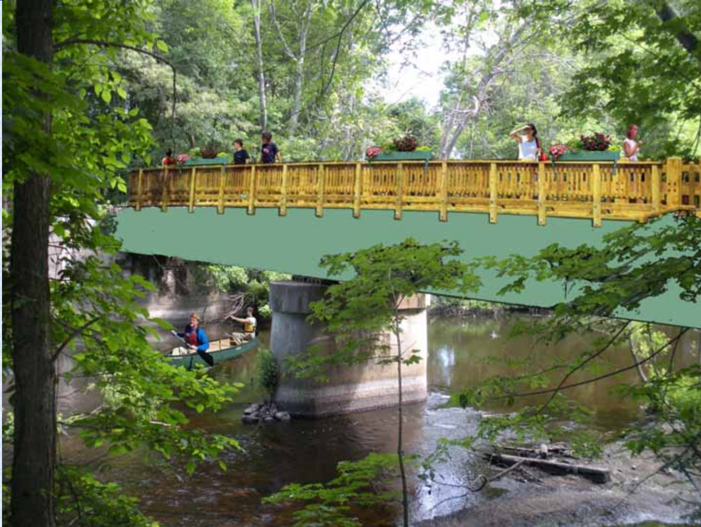
View of Charles River at renovated bridge
