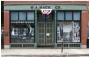
To the Mack Building In Lowell
