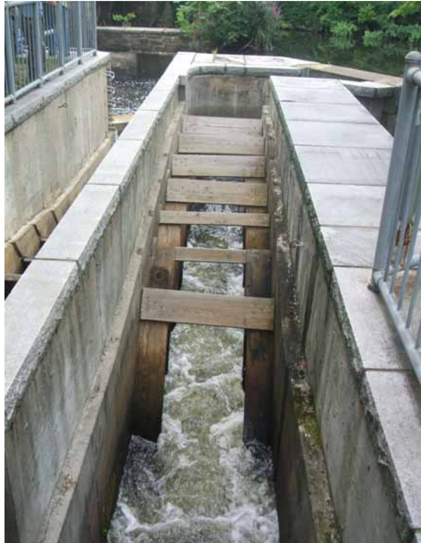
Upper Mystic Lake Dam Rehabilitation Project
