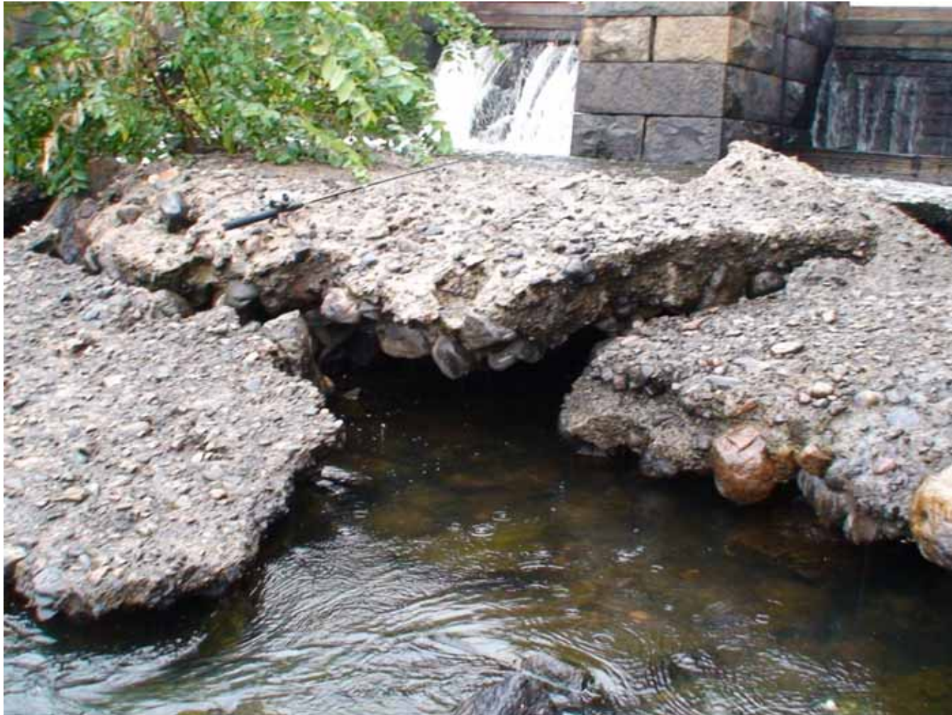
Upper Mystic Lake Dam Rehabilitation Project
