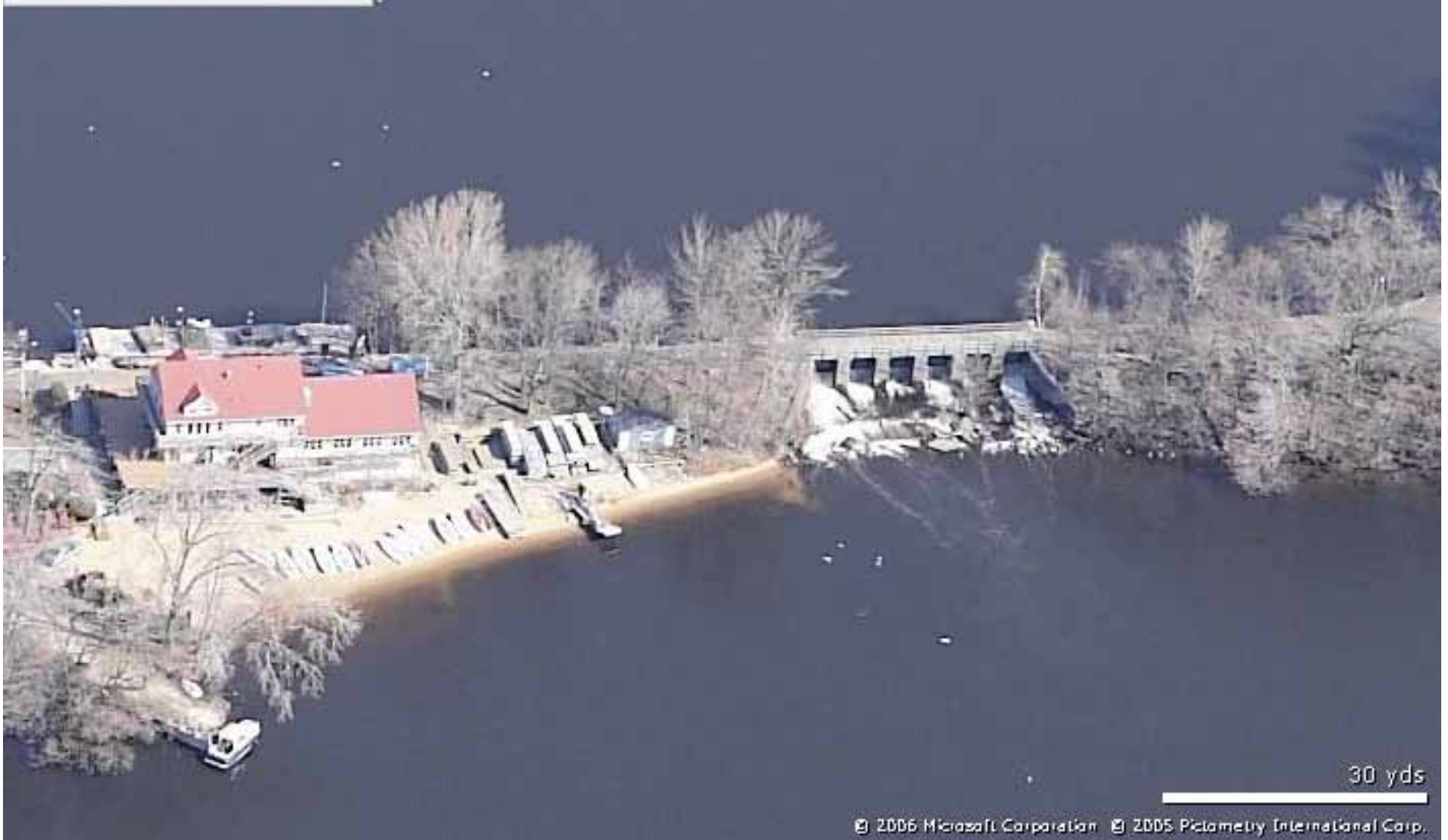
Upper Mystic Lake Dam Rehabilitation Project
