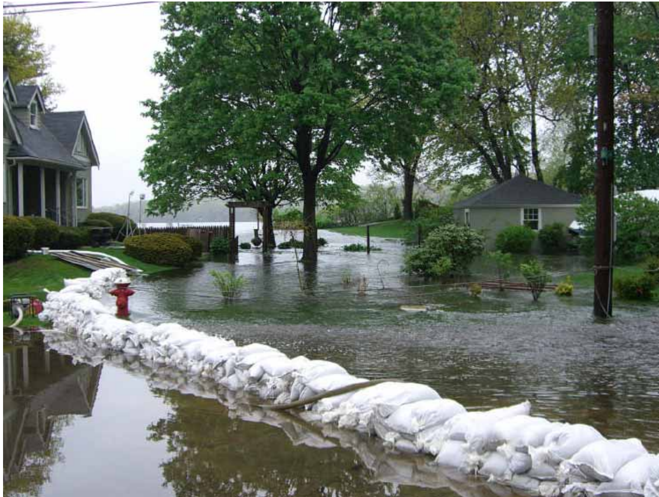
Upper Mystic Lake Dam Rehabilitation Project
