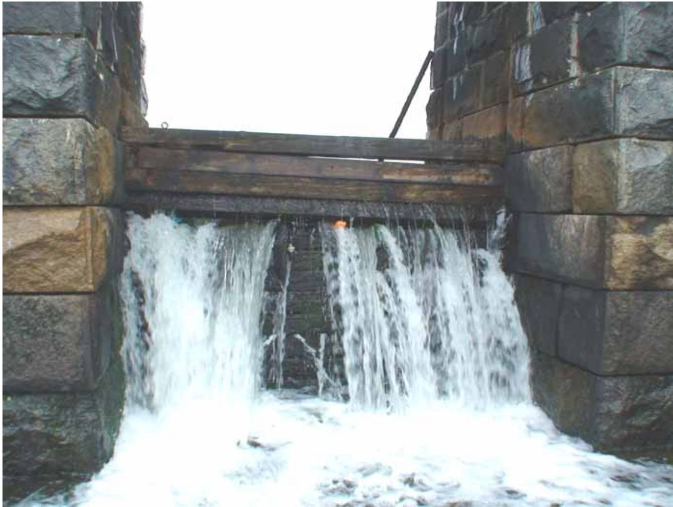
Upper Mystic Lake Dam Rehabilitation Project
