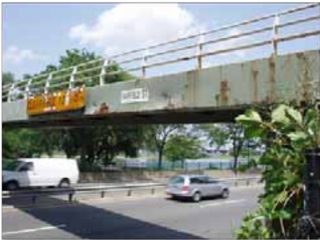
Fairfield St. Pedestrian Bridge
