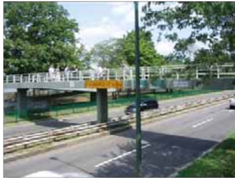
Silber Way Pedestrian Bridge
