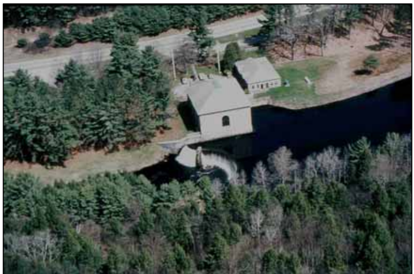
The Roger H. Lonergan Intake Works
