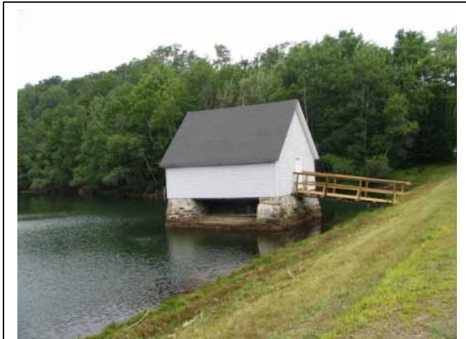
Belmont Reservoir pump house, Hinsdale, MA, Photograph by Rebekah McDermott
