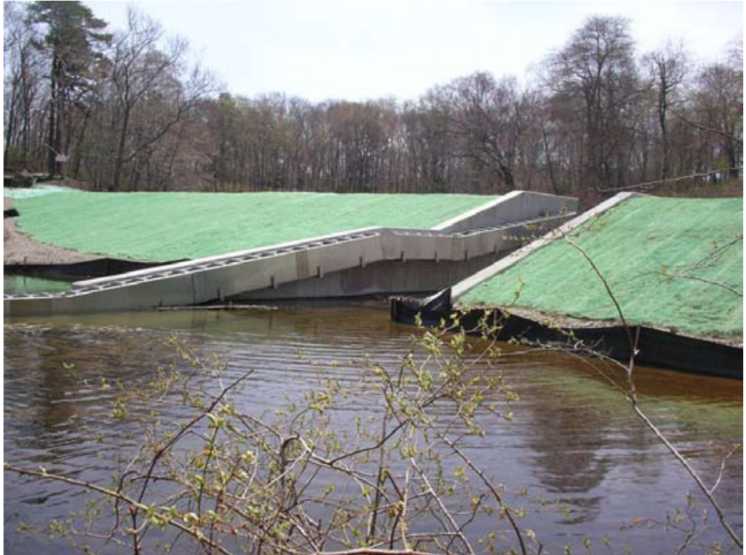
Figure 5. Alaskan Steeppass installation at Upper Shawme Pond, Sandwich, MA.
