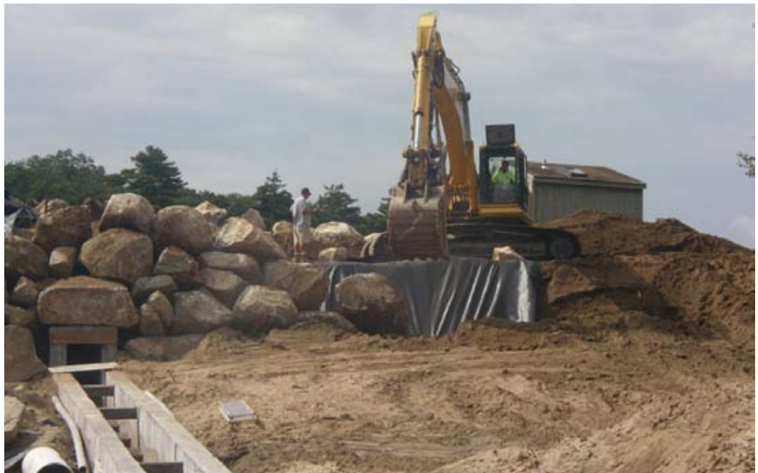
Figure 4. Russell's Millpond fishway construction, Eel River, Plymouth, MA.
