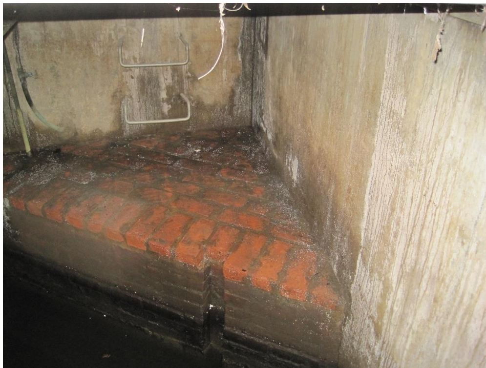
Photo 10: Wet Well Access Platform
