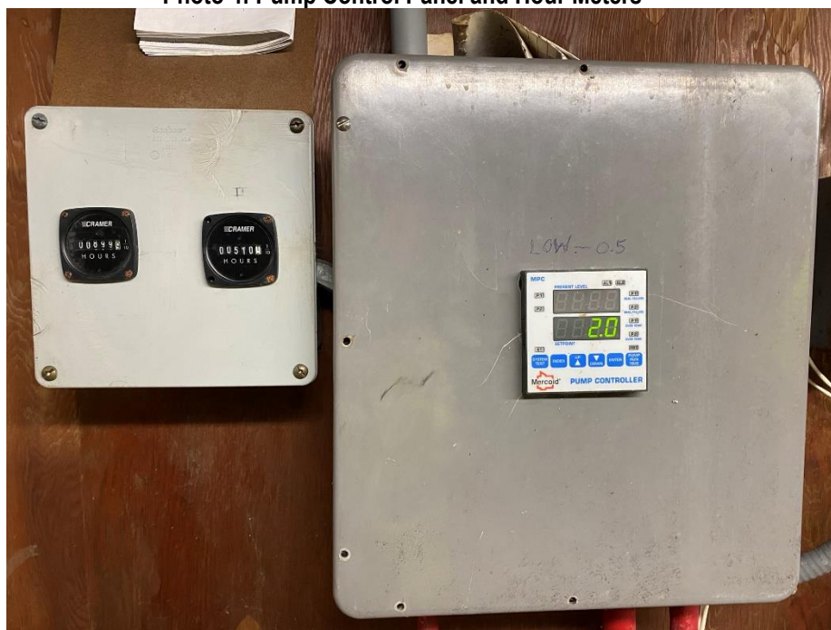
Photo 4: Pump Control Panel and Hour Meters
