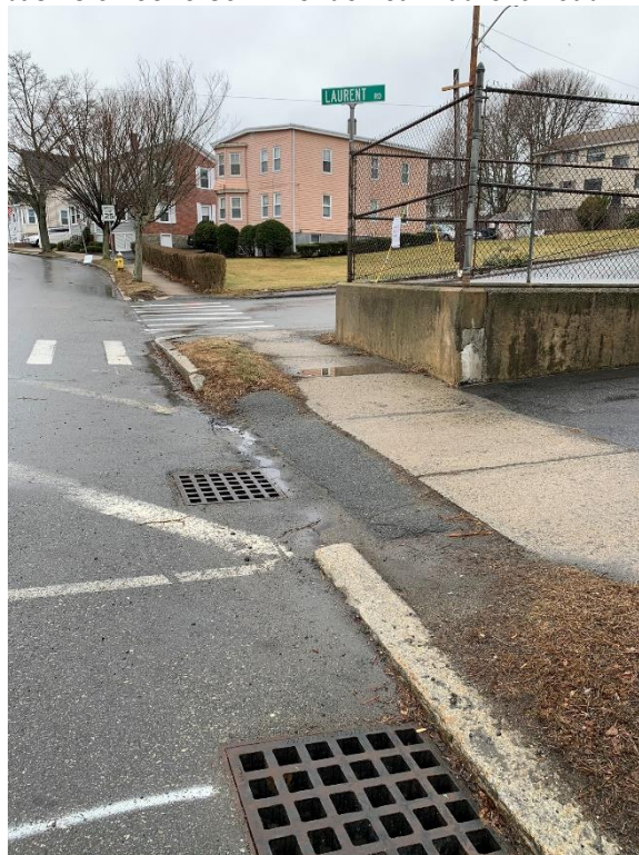
Photo 26: Catch basins on Jefferson Avenue near Laurent Road with small curb reveal.
