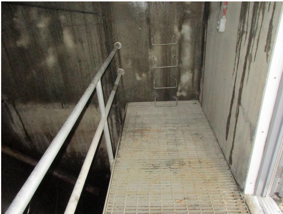
Photo 10: Wet Well Access Platform
