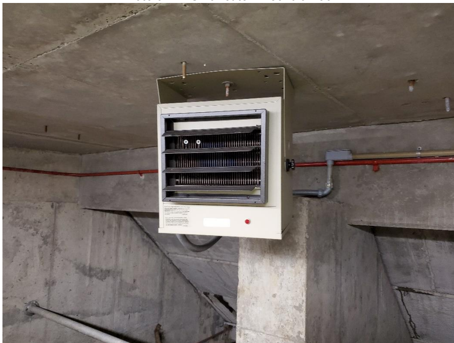
Photo 5: Unit heater in control room
