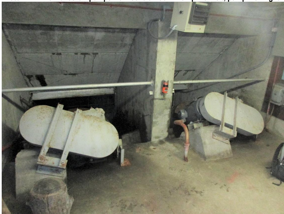
Photo 8: Screw pump 1 Gear Reducer, Motor and Upper Bearing
