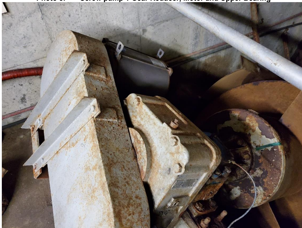
Photo 8: Screw pump 1 Gear Reducer, Motor and Upper Bearing
