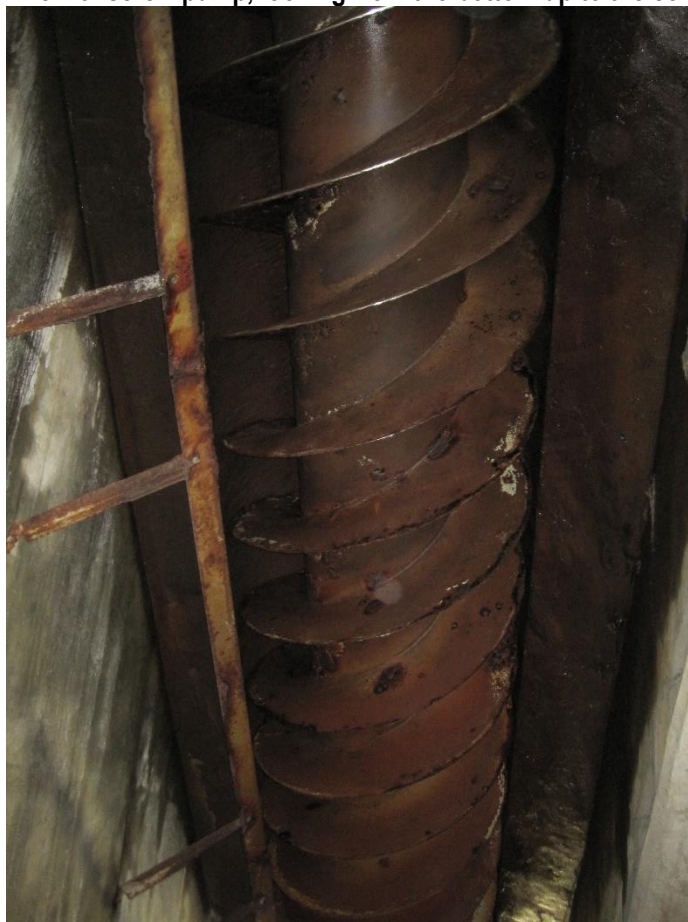
Photo 6: View of screw pump, looking from the bottom up to the control room
