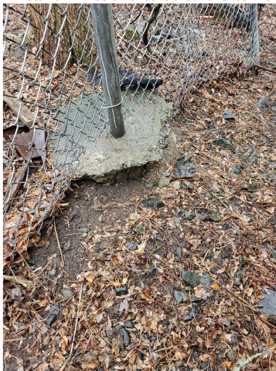
Photo 23: Erosion of soils around fence line
