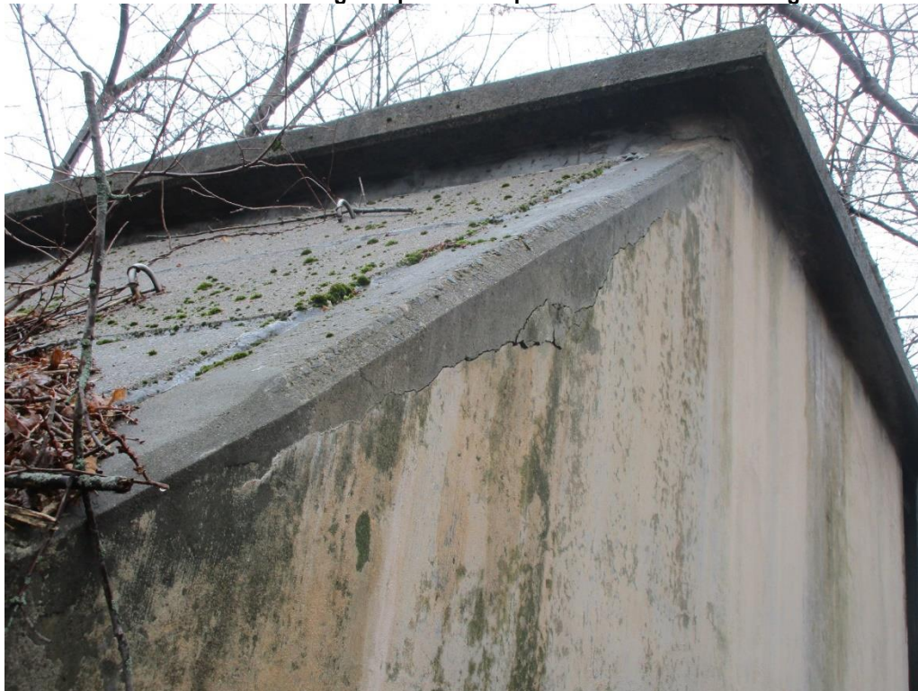
Photo 16: Cracking and previous repairs on exterior of building.
