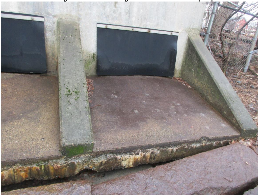
Photo 22: Displaced rip rap following discharge chute.
