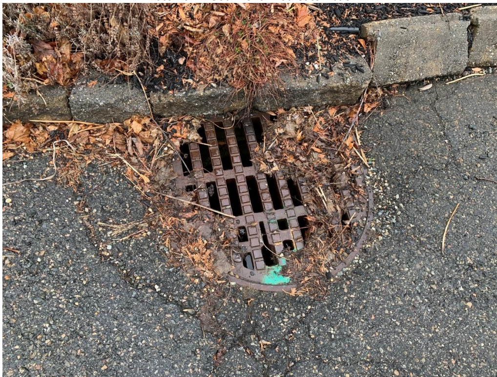
Photo 25: Sediment filled catch basin.
