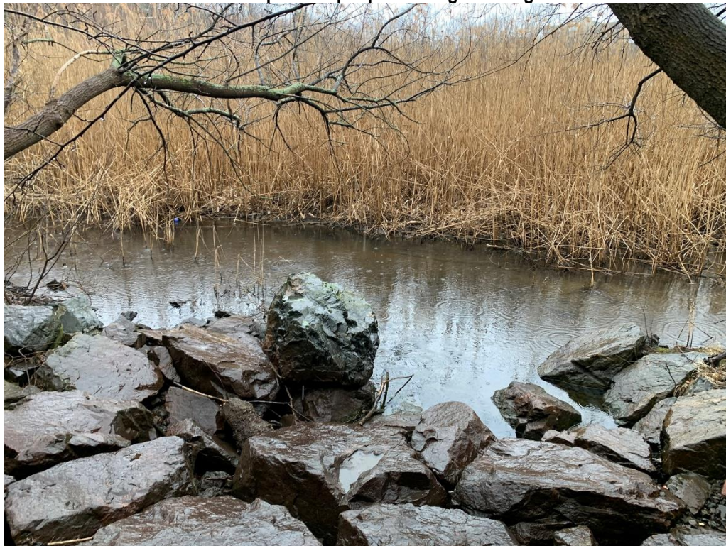
Photo 22: Displaced rip rap following discharge chute.
