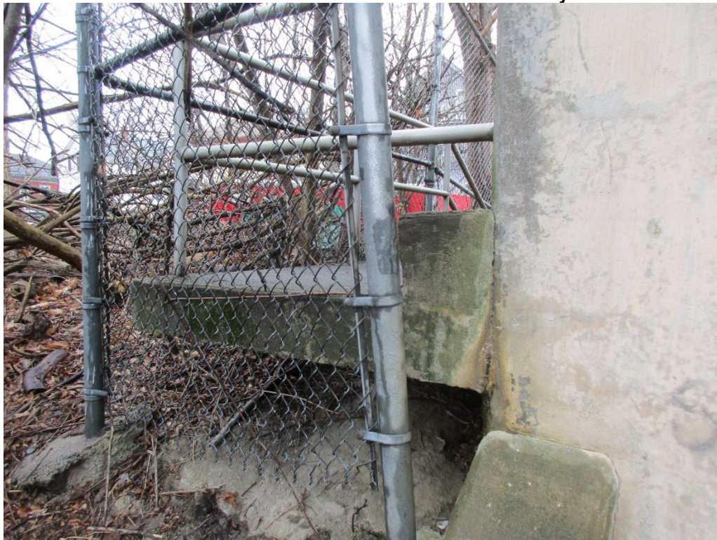
Photo 18: Soil Erosion under entrance slab and security Fence.
