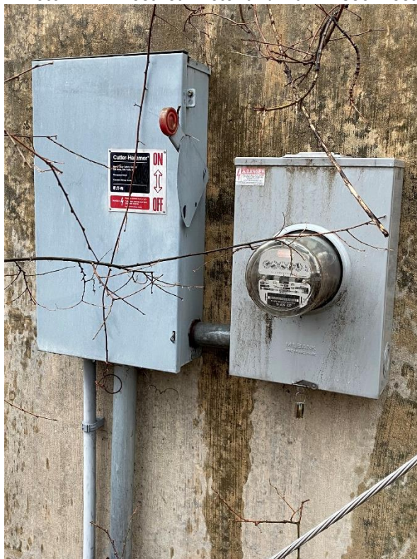
Photo 11: Electrical Meter and Main Disconnect
