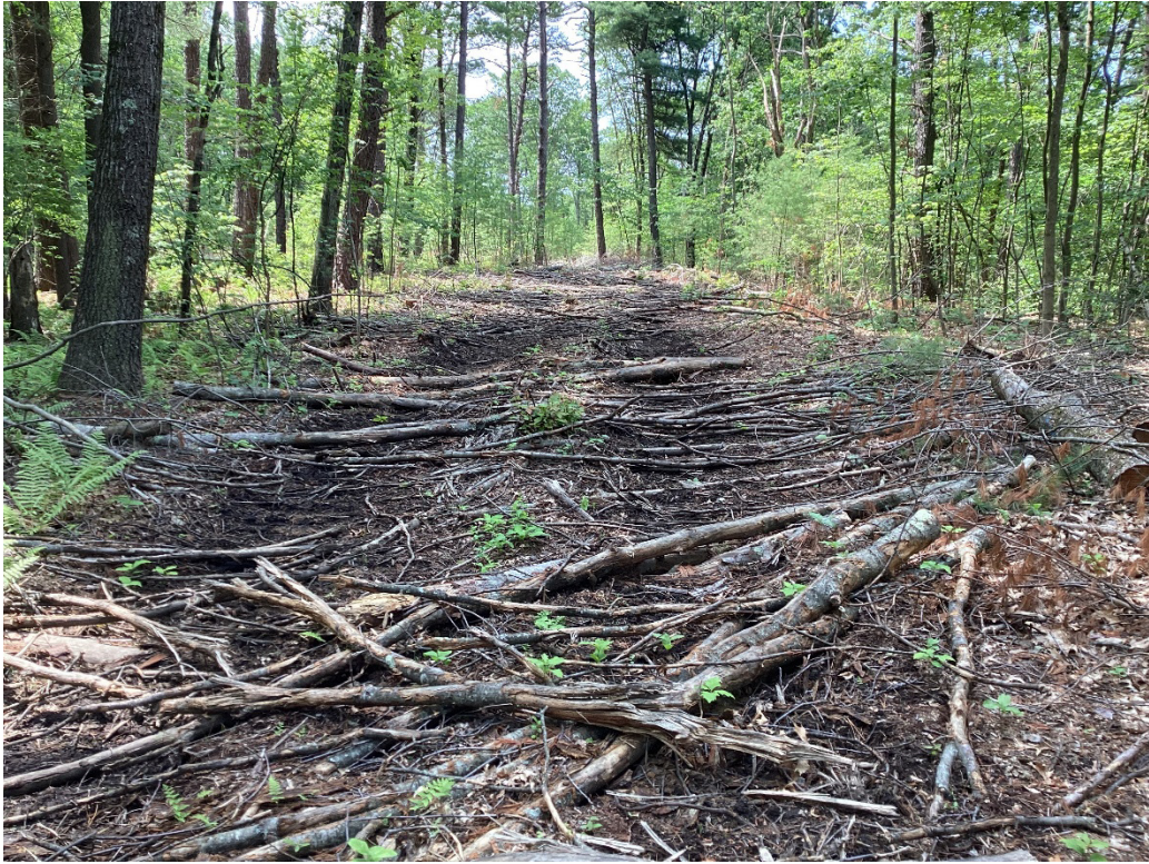
C. Tree tops and small stems were used to prevent rutting.
