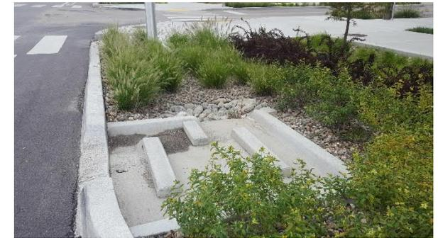
Image 3: Example of an established bioretention basin with a concrete curb cut and pretreatment structure to remove sediment before runoff enters the planted portion of the basin.
