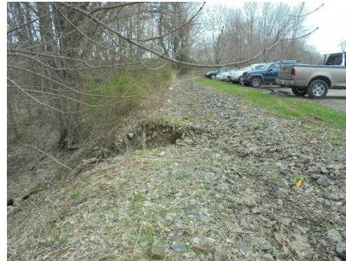
Image 2: Severe erosion at the outlet of the existing swale.
