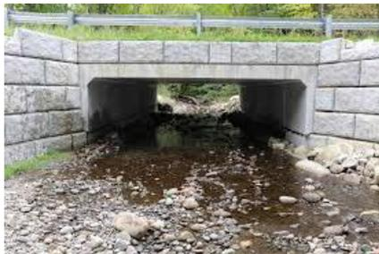
Image 3: Example of embedded box culvert (Maine Audubon).
