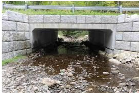
Image 4: Example of embedded box culvert (Maine Audubon).
