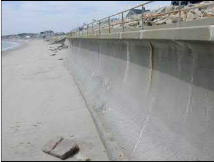
This concrete seawall was built to protect the homes and infrastructure behind it. This seawall has a curved face built into the top of the wall, which redirects some of the reflected water and waves away from the wall. (Photo: CZM)
