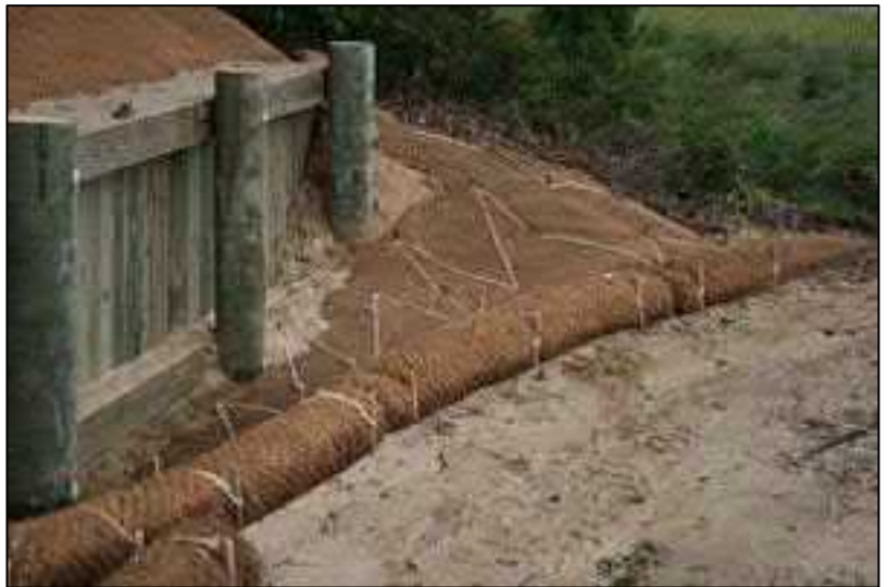
A coir roll, natural fiber blanket, and fill were installed to minimize erosion at the end of this bulkhead. (Photo: Wilkinson Ecological Design)
