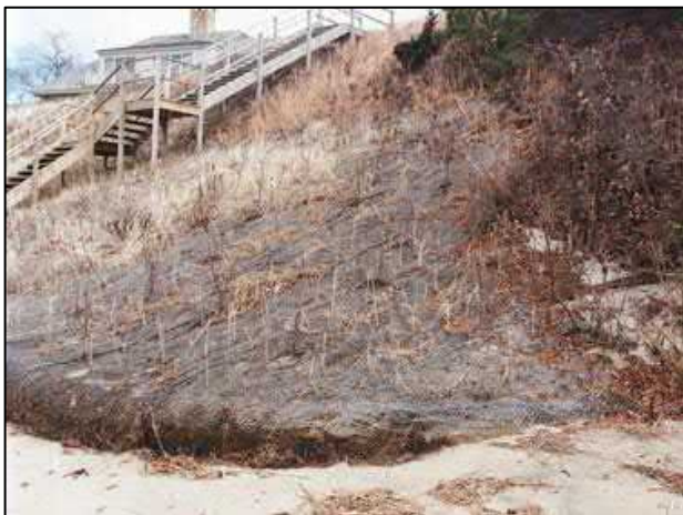
In this bank stabilization project, a natural fiber blanket was installed on the face of the bank and vegetation was planted through it. A coir roll was also installed at the base of the bank. (Photo: CZM)
