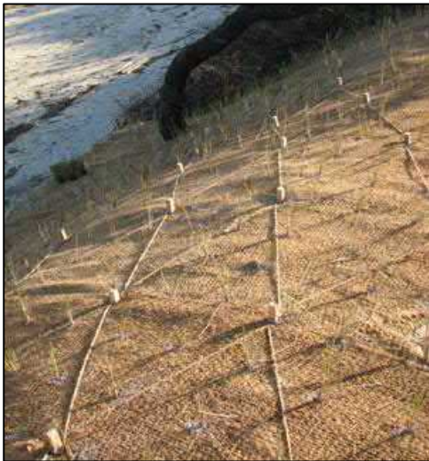
Oak stakes are used to anchor the natural fiber blanket installed on this bank. A notch in the stake is used as a stop to hold biodegradable coir twine to secure the blanket to the ground surface. Vegetation was planted through the blanket. (Photo: Cape Organics, Inc.)
