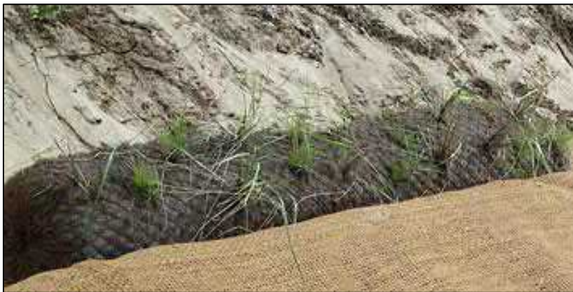
This coir roll has been planted with vegetation prior to installation. (Photo: Wilkinson Ecological Design)
