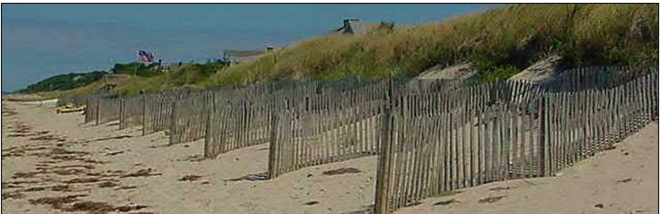
Sand fencing was installed along the base of and perpendicular to this eroded dune to trap windblown sand and help rebuild the dune. (Photo: CZM)
