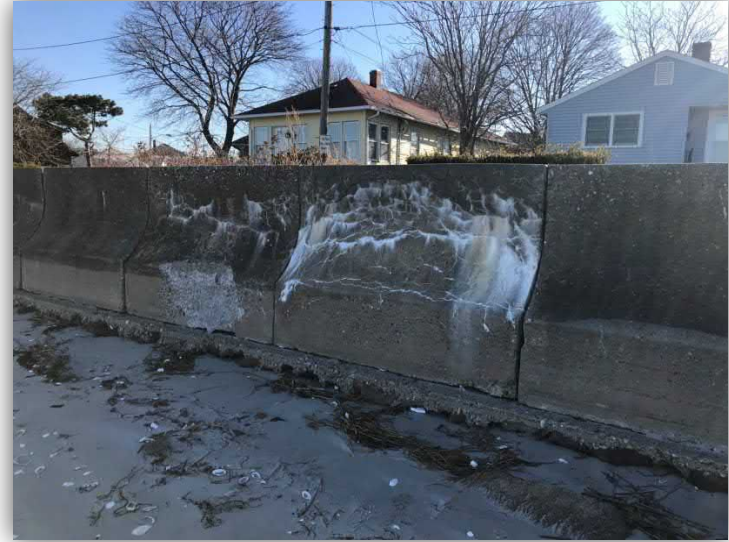
Seawall deterioration
