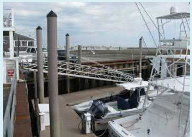
This steel bulkhead is built to hold the soil under this parking lot in place. (Photo: CZM)
