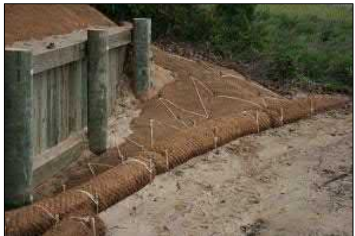
Coir rolls, natural fiber blankets, and fill were installed to prevent erosion at the end of this bulkhead. (Photo: Wilkinson Ecological Design)
