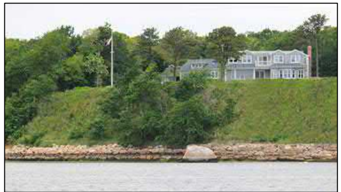
The bank above this revetment was stabilized with natural fiber blankets and native, salt-tolerant vegetation. (Photo: Wilkinson Ecological Design)
