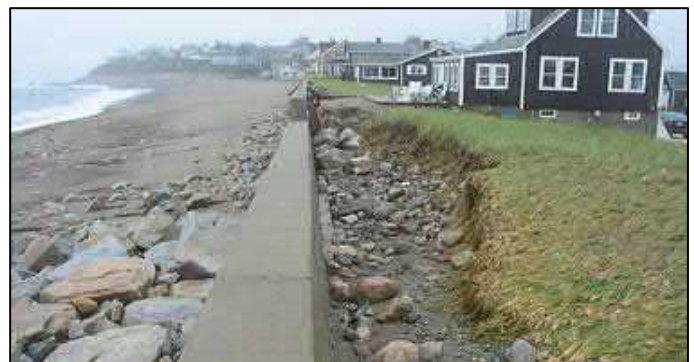
Water overtopping this seawall in a storm eroded the lawn and sediments behind it. Replacing the sediment and planting salt-tolerant vegetation may help to reduce erosion in future storms. (Photo: CZM)
