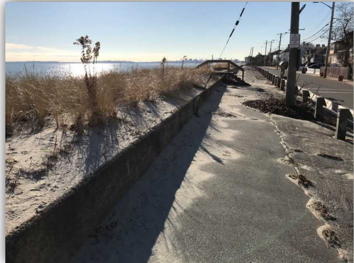
Sand overtopping seawall
