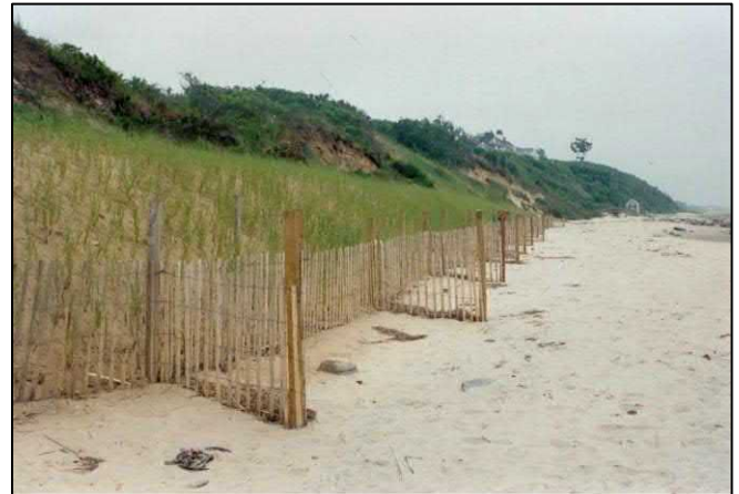
In this project, an artificial dune was built at the base of an eroding bank and heavily planted with erosion-control vegetation. Sand fencing was installed to help trap sand to build the artificial dune. (Photo: CZM)
