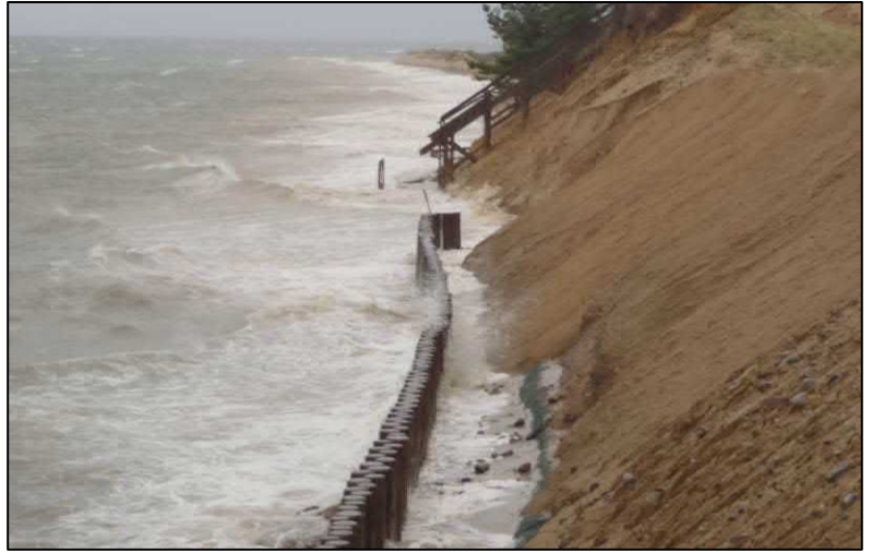
The row of posts installed at the base of this bank is acting like a solid wall, reflecting wave energy and exacerbating beach erosion and erosion of neighboring properties. (Photo: Greg Berman, Woods Hole Oceanographic Institution Sea Grant Program)
