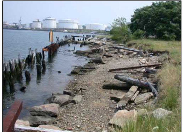
This bulkhead has deteriorated and erosion has occurred landward of it. When reconstructed, the bulkhead should be replaced with a sloping rock revetment to dissipate energy more effectively and reduce wave reflection. In addition, the toe of the revetment should be constructed at the base of the eroding bank to minimize regular interaction with waves and tides. This improved placement will reduce impacts to the beach and extend the life of the structure. (Photo: CZM)
