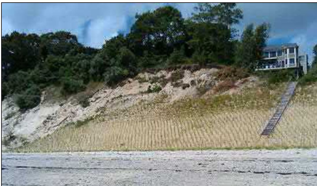
Sediment was added to this eroding bank to create a shallower and more stable slope before the vegetation was planted. The lower bank was planted with grasses and the upper section with mixed grasses and shrubs. (Photo: CZM)
