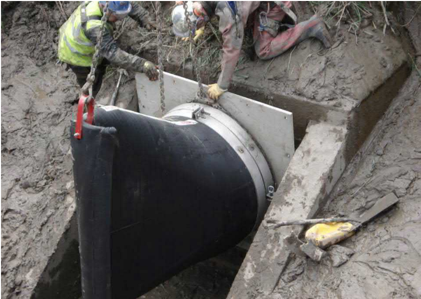
Figure 3.14 Replacement of a metal flap valve device with a duckbill backflow prevention device
