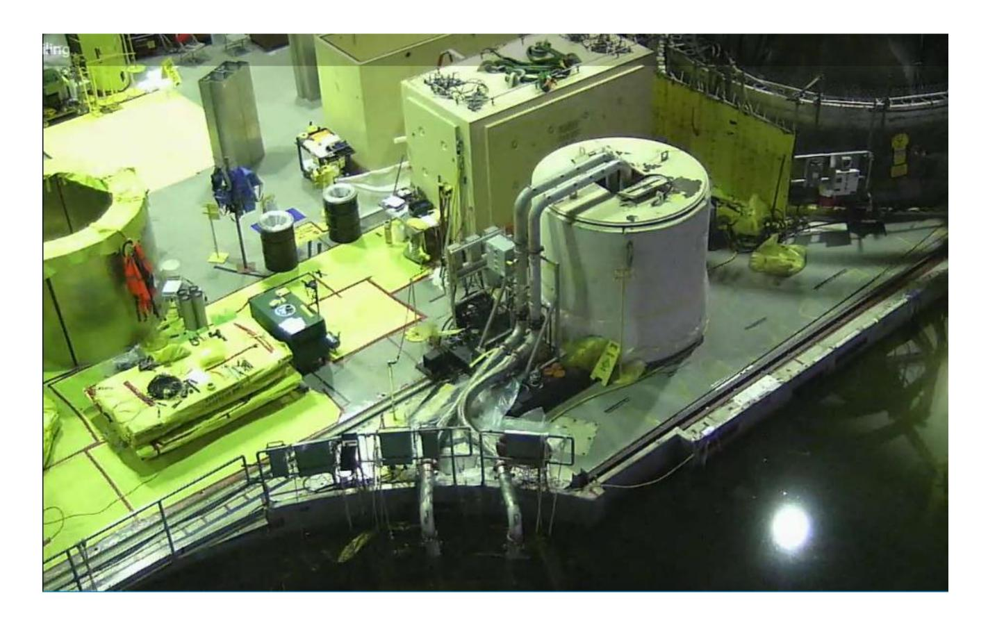
Recently installed additional advanced filtration system for Reactor Cavity and Dryer / Separator Pit. All major onsite storage volumes have dedicated high capacity / high efficiency filtration systems
