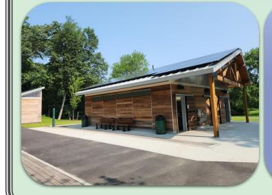
The Task Force supports net-zero goals in new construction projects. The Shannon Beach Bathhouse, completed in 2023, includes a 14kW solar array with a backup battery system to provide 100% of the facility's electricity needs.
