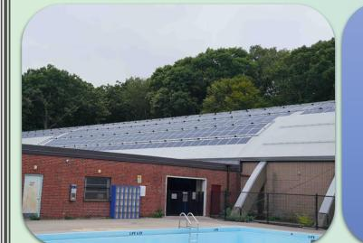
In 2022, the team identified an innovative thin-film solar PV technology that could be cost-effectively installed on barreled ice rink rooftops. Solar PV has been installed on two rinks, effectively eliminating grid electricity use. The team plans to deploy this technology on three additional sites over the next year.
