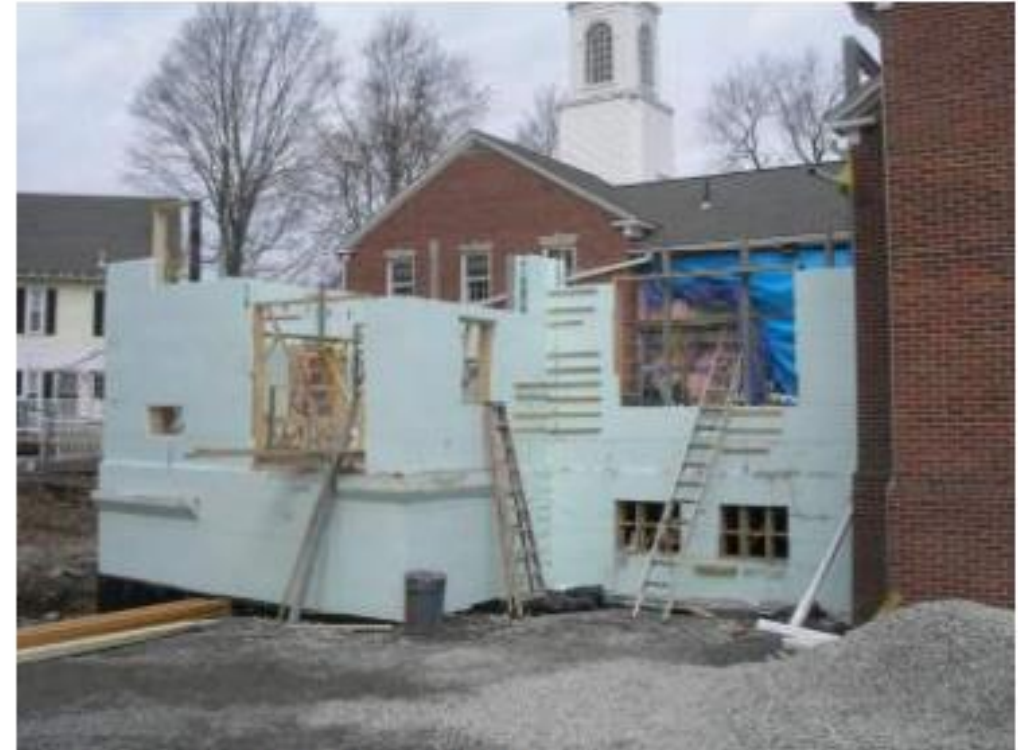
FUMC Addition: 50% slag concrete
