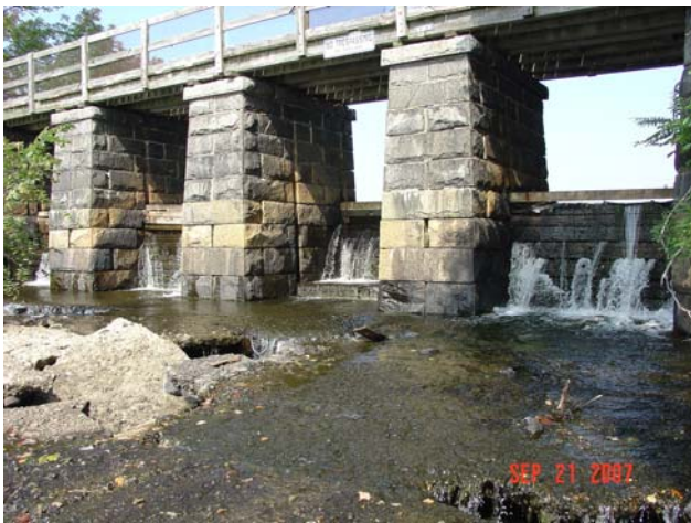
Figure 8. Mystic Lakes Dam spillway, 2007.
