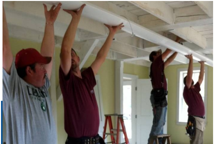
Left Photo: Workers at Appleton Farms.
