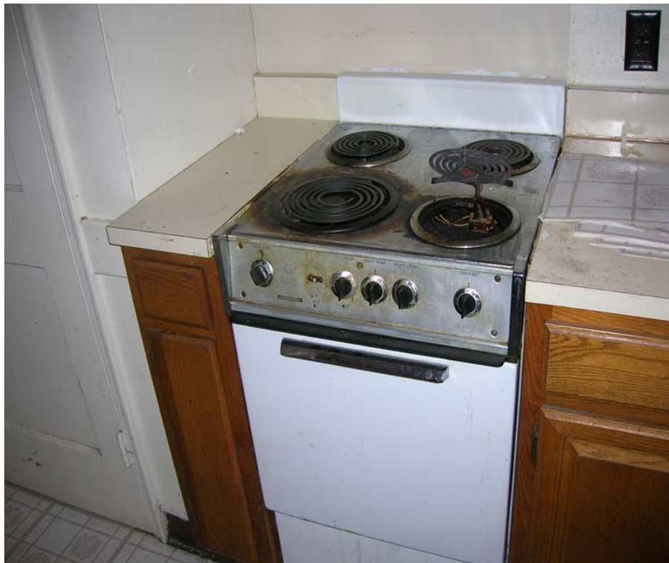
200-2 Family Housing Development, 86 Rainbow Terrace Kitchen – Stove is Filthy and Broken, Needs Replacing
