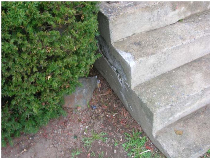
200-2 Family Housing Development, 19 Rainbow Terrace Building Exterior – Cement Stairs are Deteriorating
