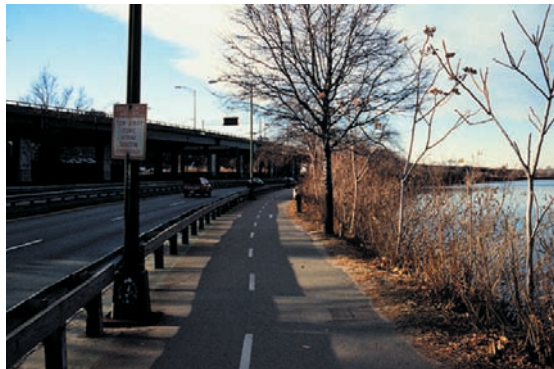
THE MASSACHUSETTS TURNPIKE (ABOVE LEFT) WALLS OFF POTENTIAL USERS IN BRIGHTON AND NEWTON FROM A SIGNIFICANT STRETCH OF THE BASIN.
