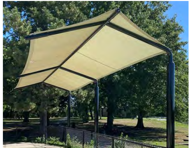
Figure C-1. Single-post / cantilever canopy at Magazine Beach (Credit: DCR)
