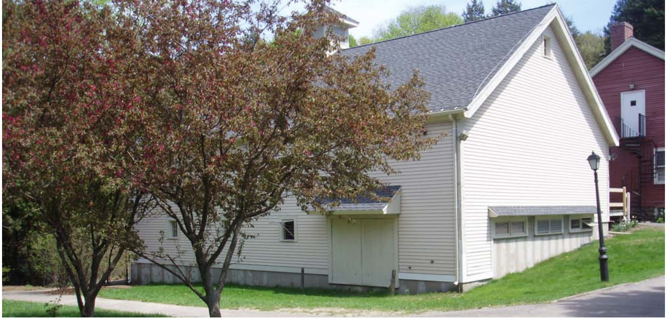
Existing Trailside Museum Lecture Wing from Canton Avenue (Pressley Associates 2007).
