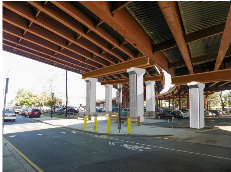
RENDERING OF TYPICAL PROPOSED SUPPORT RETROFIT
