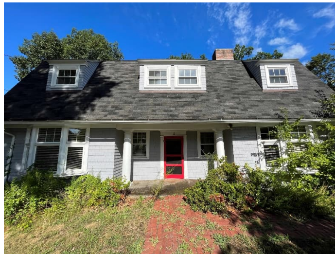
Figure 9: Existing front entrance
