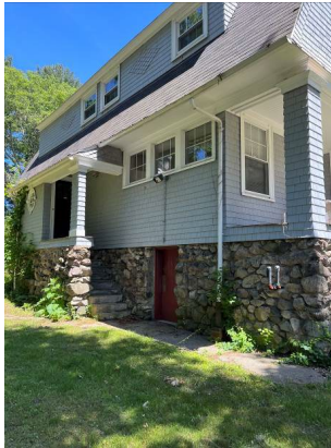
Building Mounted Lighting
