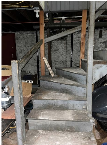
Figure 5: Winder treads in basement
