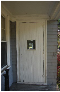
Storm Door to Deck
