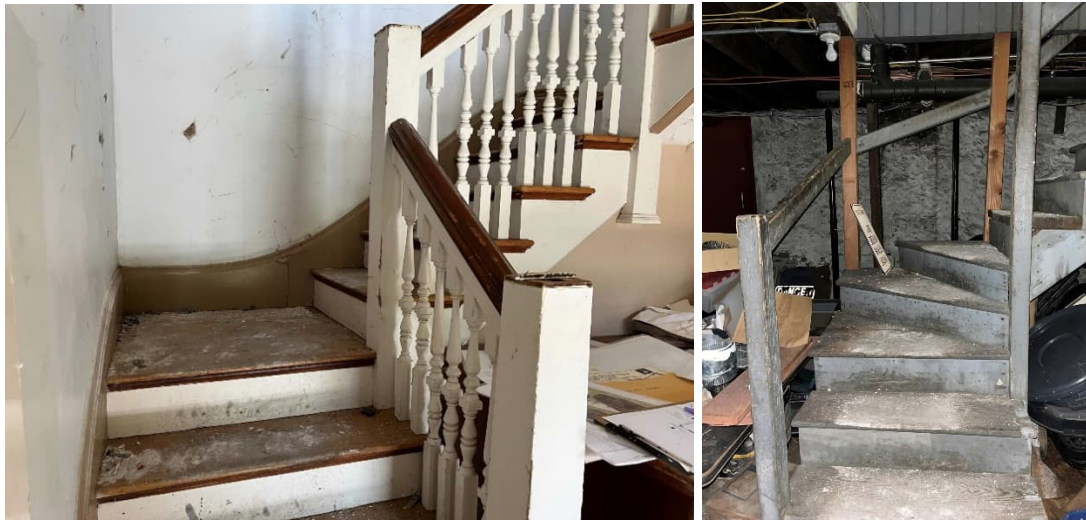
Figure 2: Handrails interrupted by newel posts
