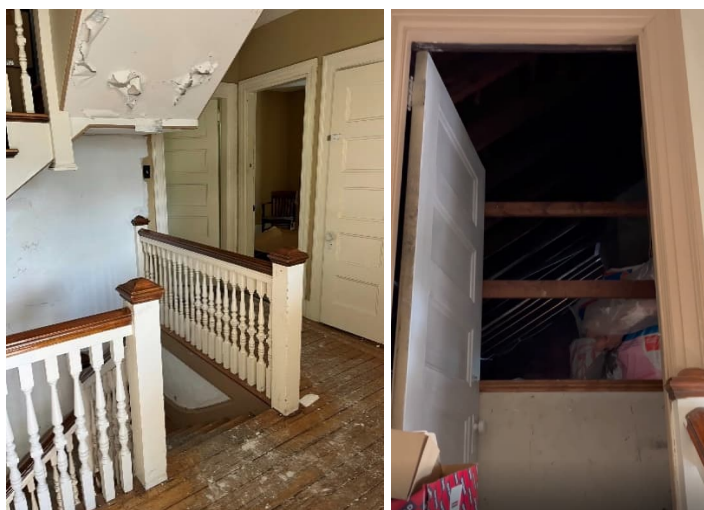
Figure 3: Low guard on Level 2 and in the Attic
