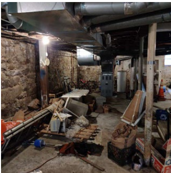
General view of basement
