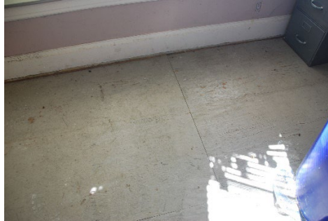
First Floor Dining Room: Plywood Subfloor
