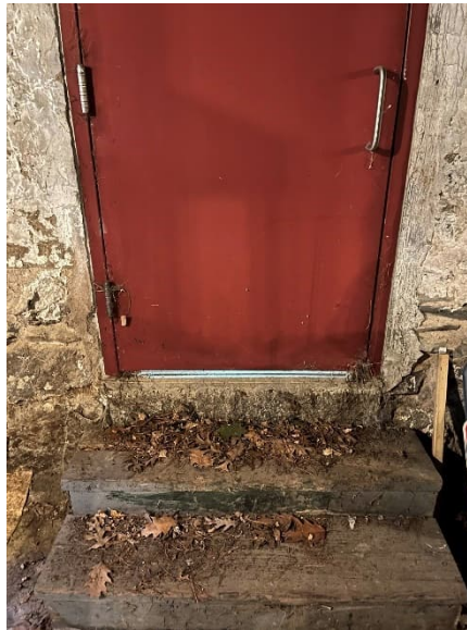
Figure 6: Steps at basement exterior door
