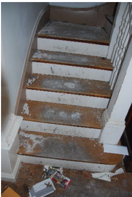
General Condition of Stair
