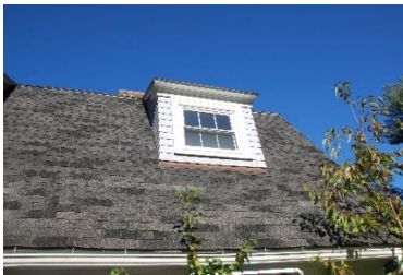
Asphalt Shingle Roof
