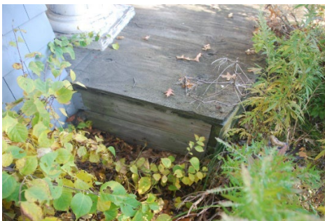
Plywood deck at Entry
