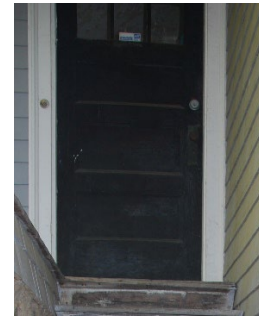
Rear Stairs at Kitchen
