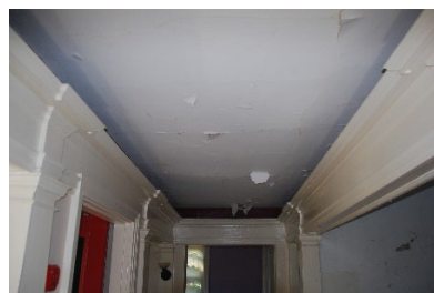
Ceiling at Front Hall
