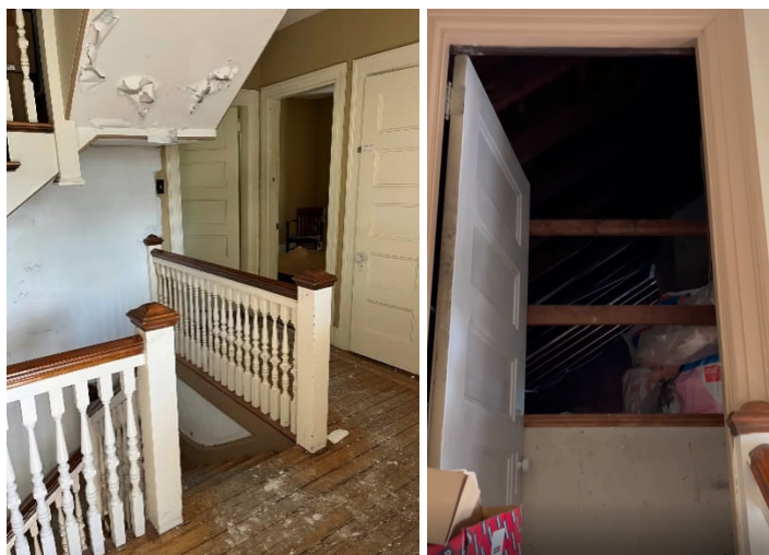
Figure 4: Low guard on Level 2 and in the Attic
