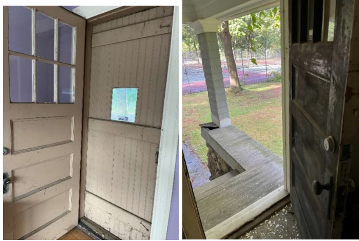
Figure 10: Non-compliant doorknobs
