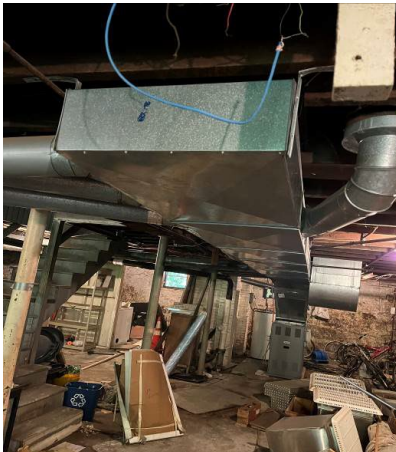
Uninsulated Ductwork
