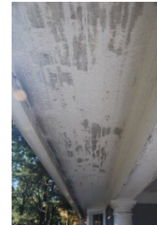
Paint at Soffit
