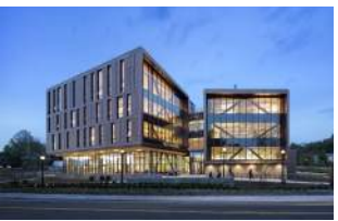
UMass Amherst Design Building Amherst, MA LEED Gold
