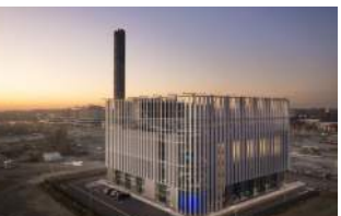
Harvard University District Energy Facility Allston, MA LEED Gold
