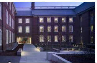
Brown University Metcalf Hall Renovation Providence, RI LEED Gold
