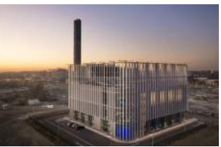
Harvard University District Energy Facility Allston, MA LEED Gold
