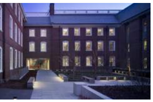
Brown University Metcalf Hall Renovation Providence, RI LEED Gold
