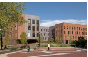
University of Connecticut Oak Hall Storrs, CT 2nd LEED Gold Certified new building for UConn
