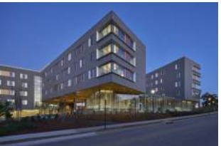
Adohi Hall University of Arkansas Fayetteville, AR LEED Silver v4
