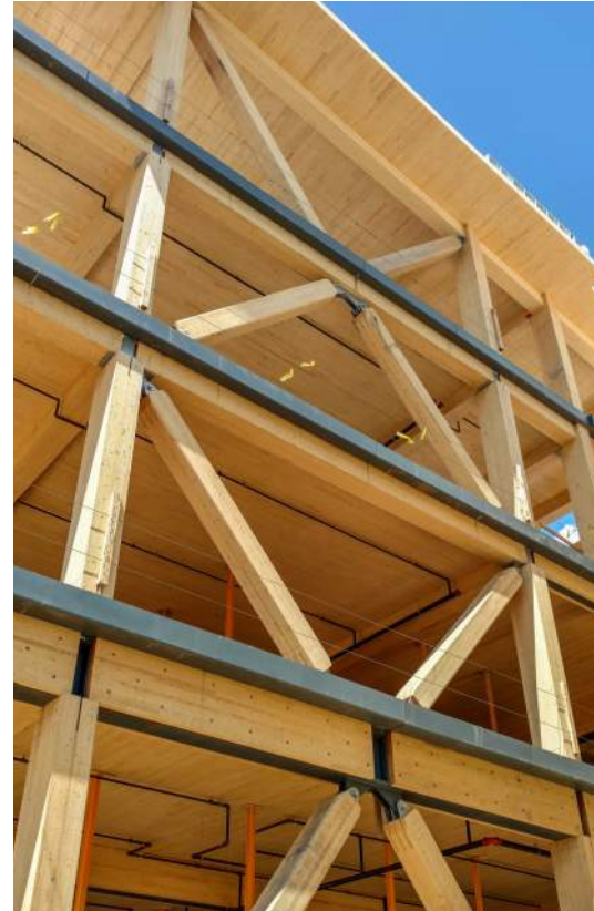
Construction detail at John W. Olver Design Building
