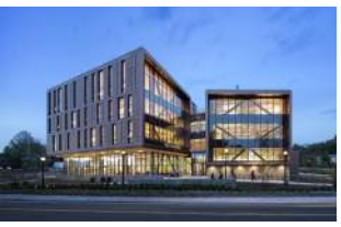
UMass Amherst Design Building Amherst, MA LEED Gold
