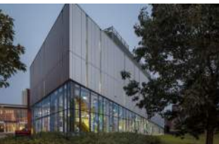
North Chiller Plant UMass Amherst LEED Silver
