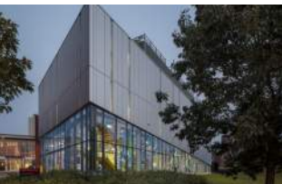
North Chiller Plant UMass Amherst LEED Silver
