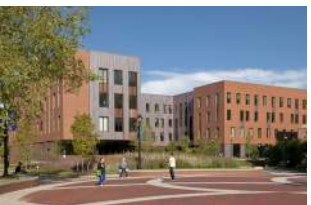
University of Connecticut Oak Hall Storrs, CT 2nd LEED Gold Certified new building for UConn
