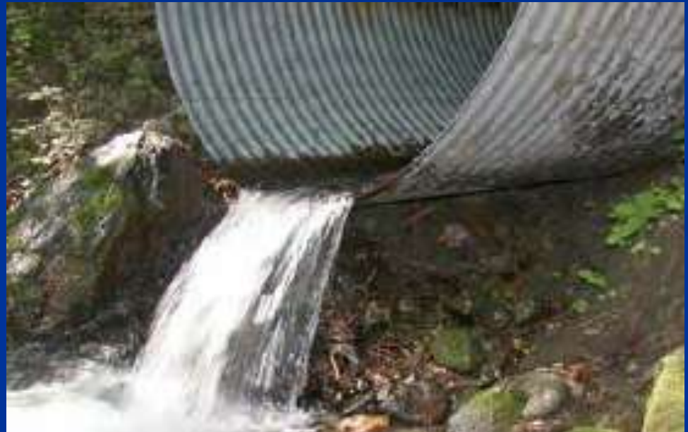
Perched Culvert, courtesy of MA Riverways Program
