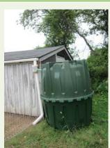
From there the rainwater from each tank could be pumped into a large 2,400 gallon tank and into the irrigation system for their fields. This collection system is able to collect over 800 gallons of water from a ½ inch rainfall event. Based on their town's rainfall, this represents over 80,000 gallons of water saved annually.
