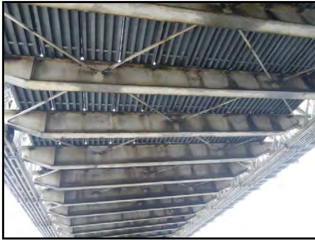
Figure 2-17 Typical Failure in Galvanized Coating
