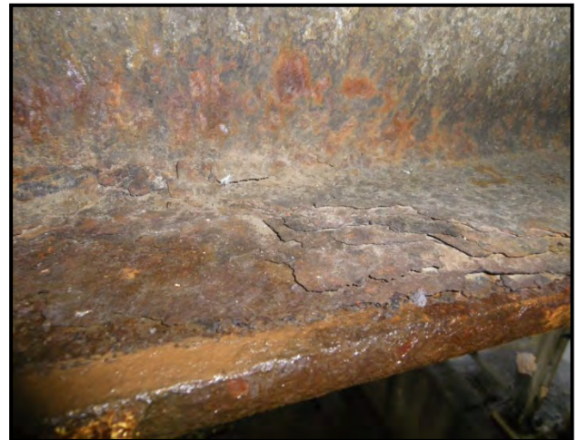
Figure 2-19 Sheared Bolt at the End of a Transom
