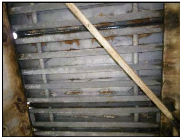
Figure 2-13 Typical Deck Panel Condition
