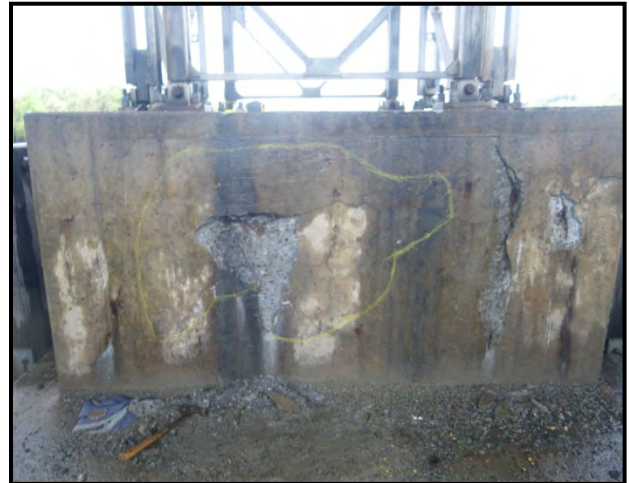
Figure 2-21 West Concrete Pedestal at Pier 3
