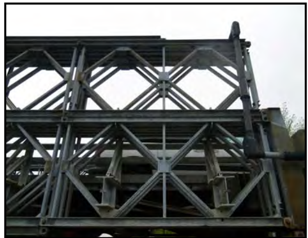
Figure 2-18 Beginning of Lamination/Section Loss
