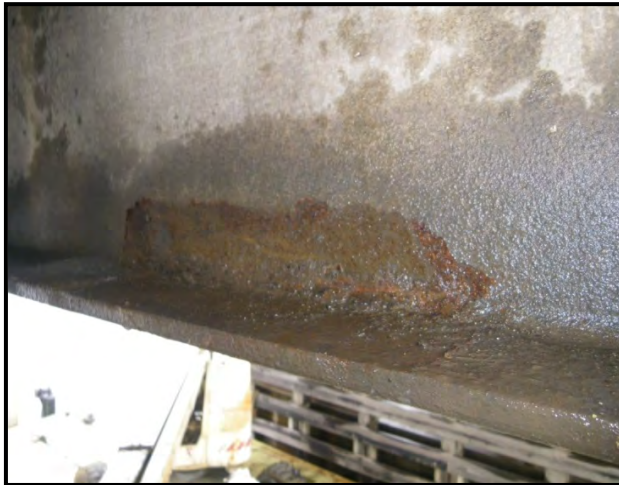
Figure 2-17 Typical Failure in Galvanized Coating
