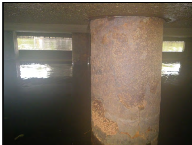
Figure 2-22 Typical Steel Pile with Moderate Rusting
