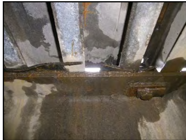
Figure 2-14 Loose Deck Connection, Broken Neoprene
