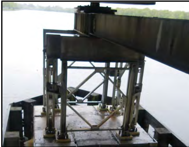
Figure 2-20 Typical Acrow Panel Tower
