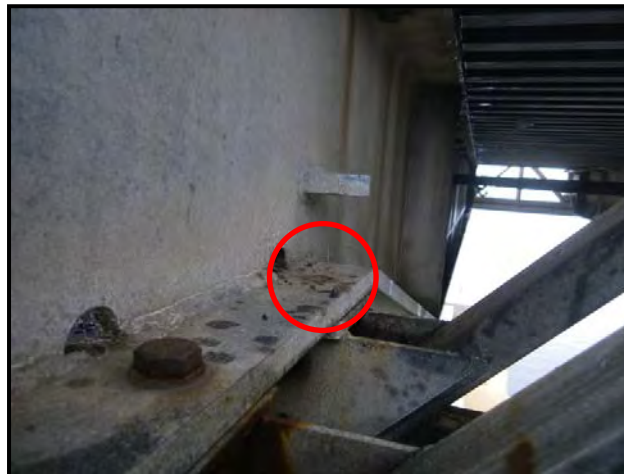
Figure 2-19 Sheared Bolt at the End of a Transom
