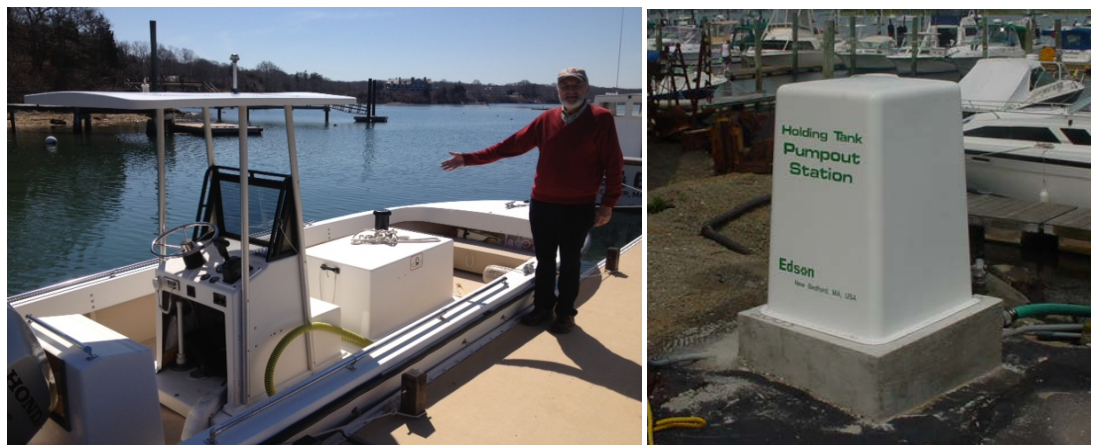
Figure 53. A combination of pumpout boats (left) and fixed location pumpout stations (right) help meet the needs of the Commonwealth's recreational boaters.
