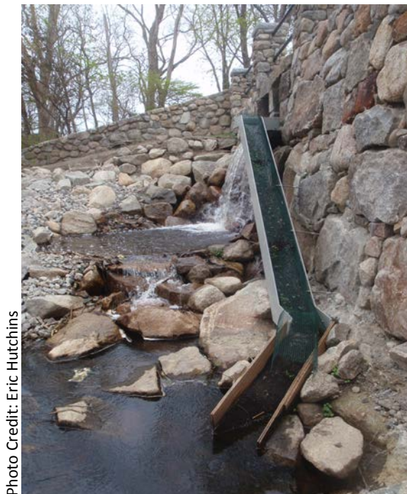
Figure 51. Eel ramps in coastal rivers provide eel passage over barriers.
