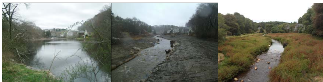
Figure 19. The Off-Billington Street Dam Removal Project: on the left is the impoundment prior to dam removal in April 2013; in the center is the drained impoundment and engineered stream bed in April 2014; and on the right is the stream in September 2014 after one full growing season. Over $122,000 in ILF funds were used for vegetating the embankment created when impoundment upstream of dam was removed.
