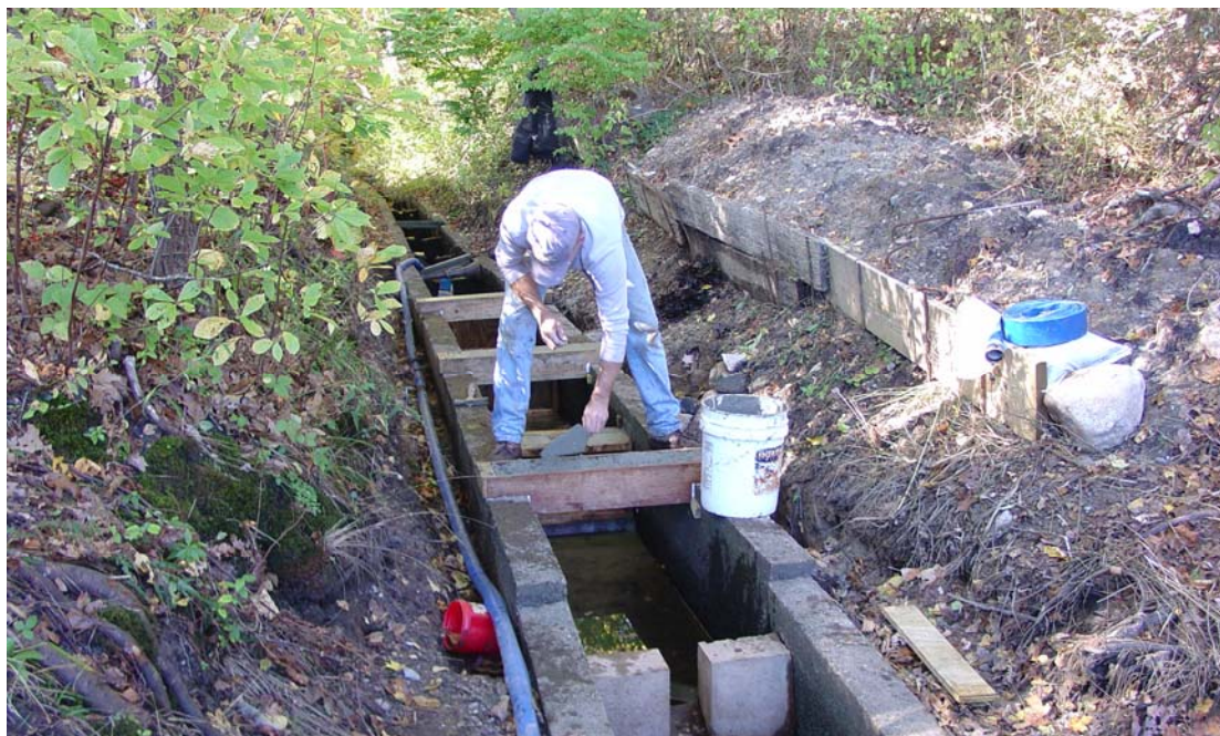
Figure 48. MarineFisheries' Edward Clark works on repairs to a degraded concrete weir and pool fish ladder in Orleans between Pilgrim Lake and tidal waters.
