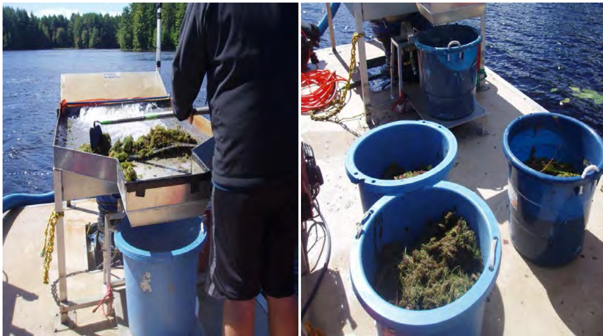
Photo shows plants collecting on double mesh screens. Water flowed back into the Regulating Pond as vegetation was pulled into buckets for safe disposal.
