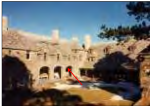
Cavity fill – Masonry/Plaster Conditioned space above covered outside walkway
