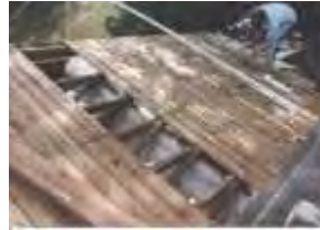
Inject closed roof slopes
