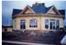
New construction – outside
