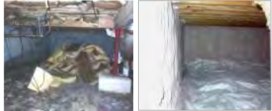
Crawl space – before and after mitigation work
