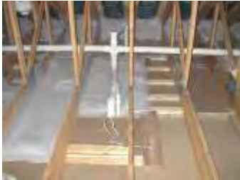
SPF for air sealing in attics before installing fiber insulation
