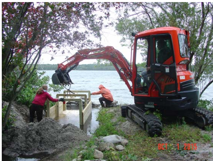
Figure 42. Installation of a new fishway at Seymour Pond.
