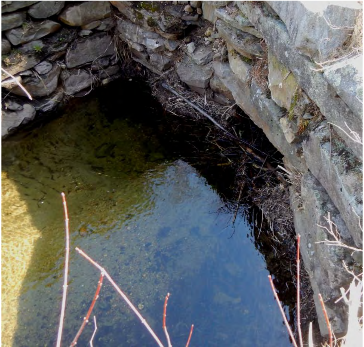
Photo 2. Upstream side Gate 22 road culvert - fresh nip twigs and debris.
