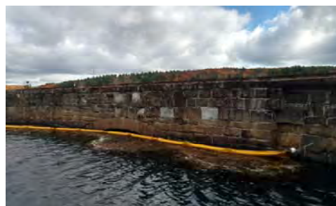
Figure 29: Fragment barrier installed at Quinapoxet Basin railroad bridge.
