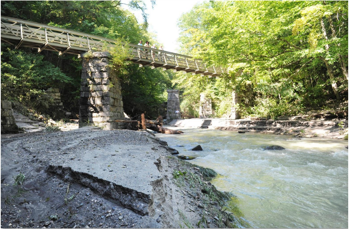
Top hazards identified by the workshop participants include heavy rains and flooding such as when the South River, at the Conway Station foot bridge, was scoured and parts of the riverbank washed away at the height of flooding during Tropical Storm Irene.
