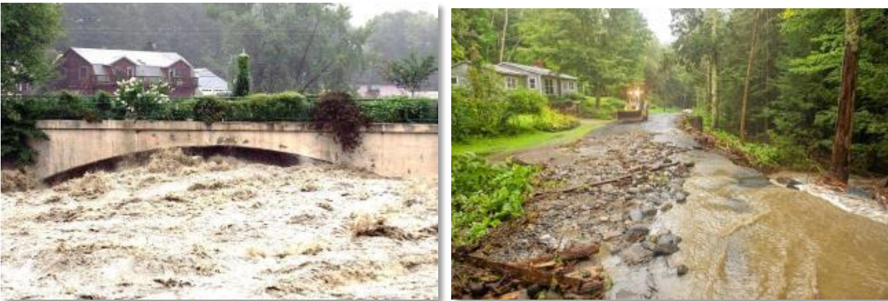
Tropical Storm Irene, with widespread flooding, foreshadows the types of extreme weather events predicted to be more prevalent in the coming years, impacting waterbodies in Town, including the Deerfield River (left) and Clesson Brook (right).
