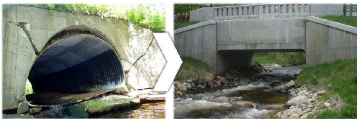
Figure 2.7 Example of Culvert Replacement
