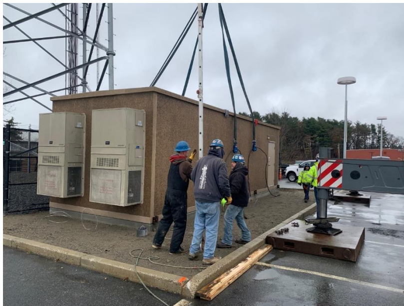
Image 16: Shelter placed on footing by crane
