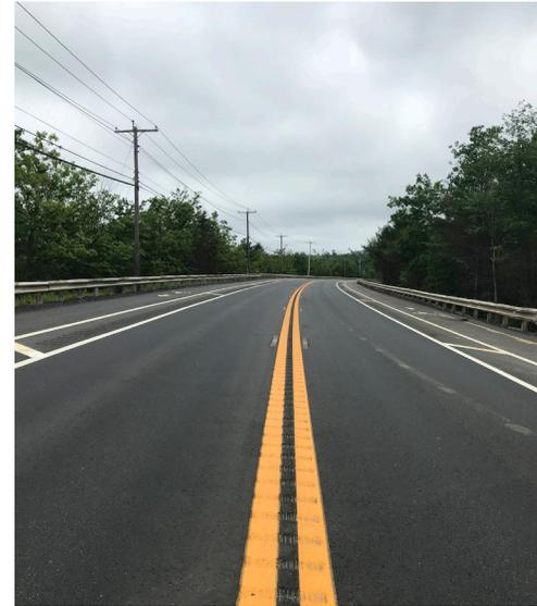
MassDOT implemented buffered bike lanes along Route 20 in Brimfield as part of a routine resurfacing project.
