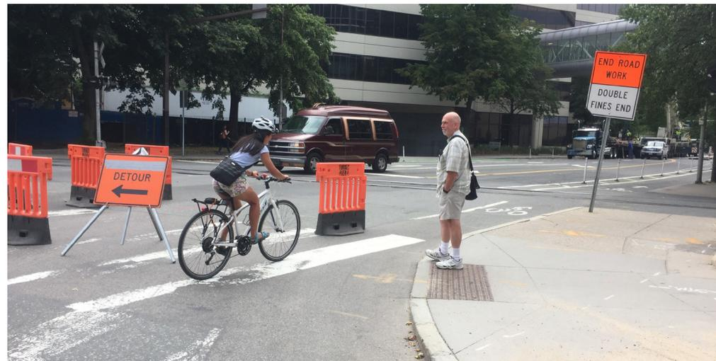
Bicyclists are sensitive to detours. Where feasible, provide a bike route through construction zones, even if access is restricted for motor vehicles, as shown.
