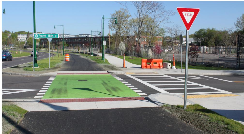
A two-way bike crossing under construction as part of the Casey Arborway project. This bike crossing features green colored pavement and is adjacent to a separate high-visibility pedestrian crossing.
