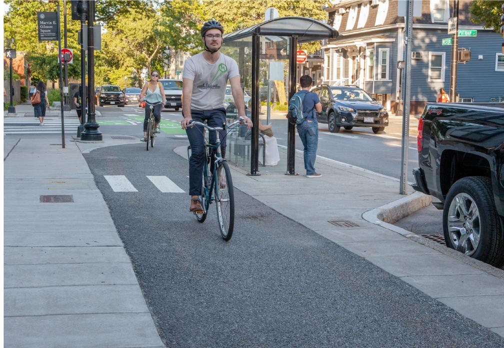
A floating bus stop implemented on Western Avenue, Cambridge. A 12' offset between the separated bike lane and bus shelter is recommended to reduce the risk of handlebar strikes. The glass shelter and clutter-free design of this floating stop ensures that pedestrians crossing the bike lane are visible to bicyclists.
