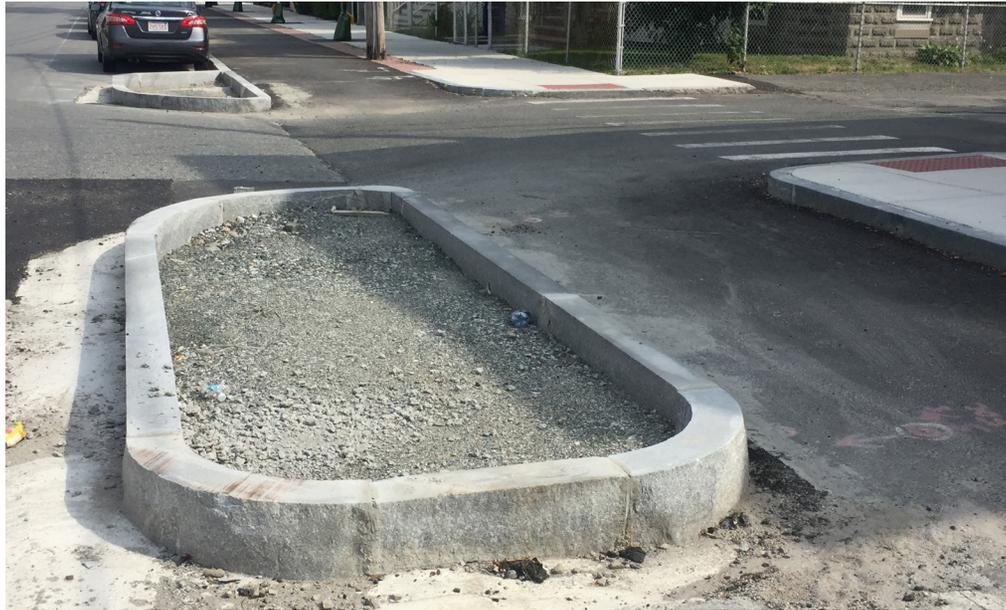
Incorporating protected intersection design principles does not always require the intersection of two separated bike lanes. For example, these under-construction corner islands where a separated bike lane intersects a side street will improve visibility for all modes and create crossing islands for people walking.
