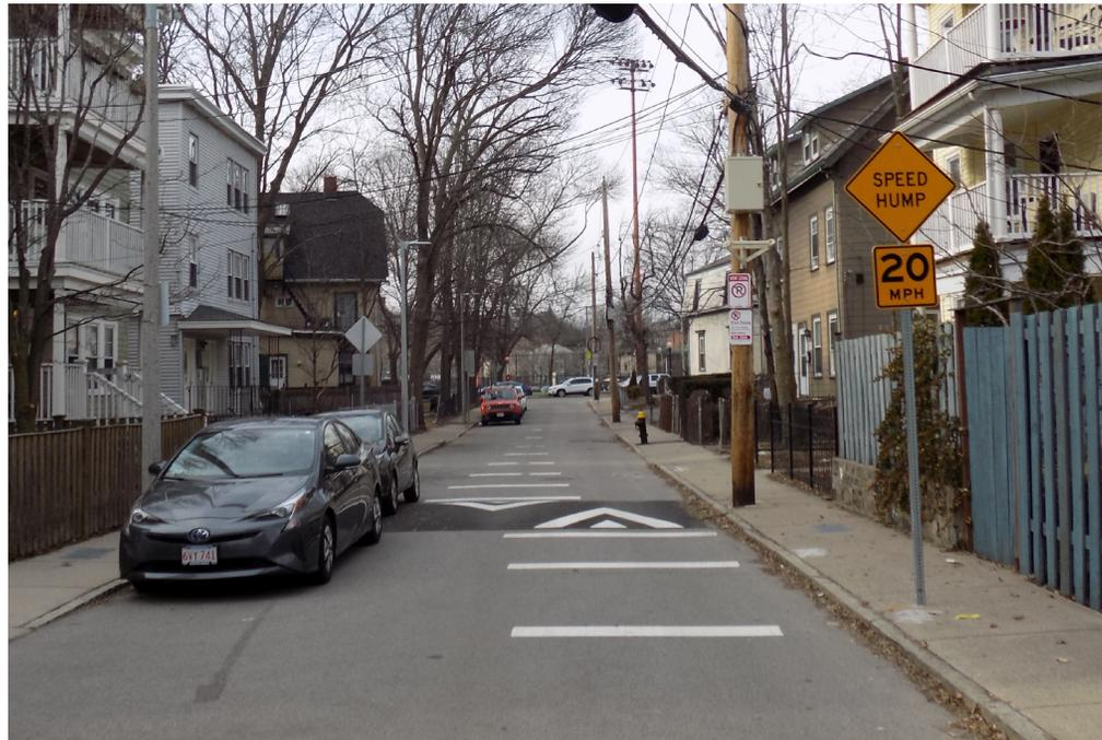
Bike boulevards are characterized by the use of traffic calming measures to reinforce 20 mph or lower operating speeds.
