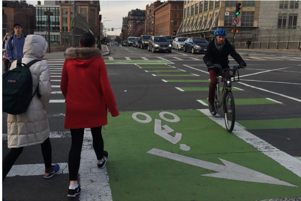
A two-stage turn queue box located between a pedestrian and bike crossing in Back Bay, Boston.
