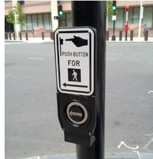
Example of an accessible pedestrian signal.
