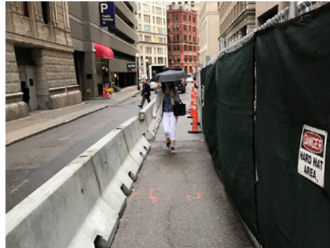
Figure 20. A temporary walkway separated from traffic through a construction zone
