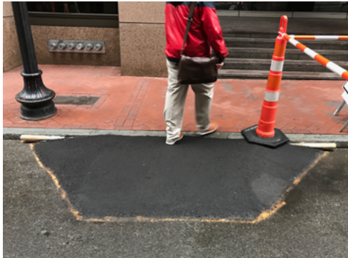
Figure 19. An example of a temporary accessible curb ramp in a construction pedestrian detour
