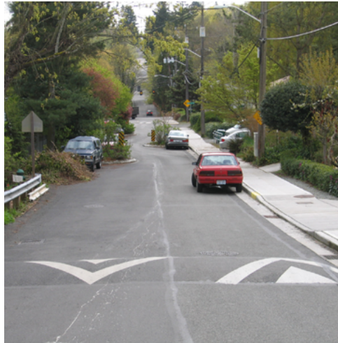
Figure 17. Speed humps, shown here on a residential street, are a traffic calming strategy.
