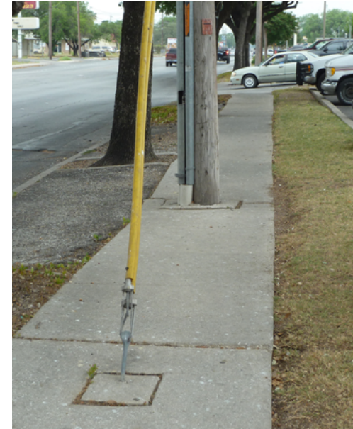
The placement of utility poles and signs can become obstacles and create accessibility challenges for people with disabilities.
