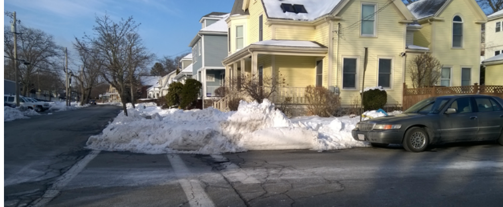
Snow plows should not pile snow on crosswalk curb ramps.
